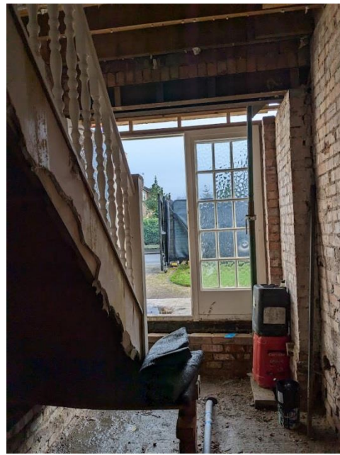
Photograph 12. Front, ground floor entrance
