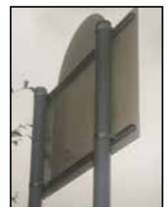
V9. Channel and posts.
