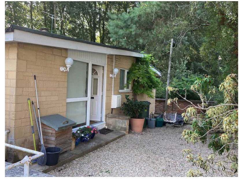
View of NE elevation (location of proposed extension)
