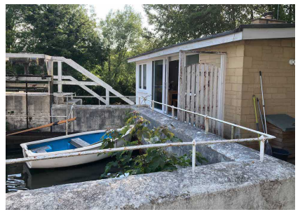
Flood protection wall surrounding property
