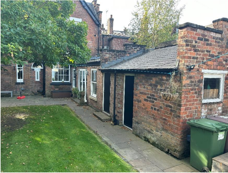
Existing Photograph of single storey outrigger to be extended.
