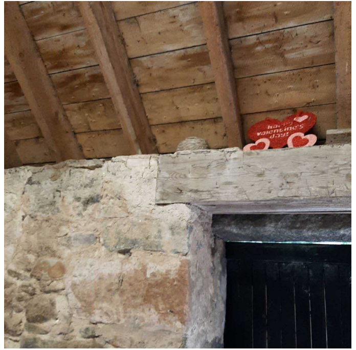
Timbersafe lintel in good condition
