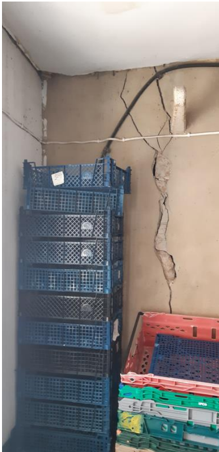
Settlement Crack Barn 1 SW Corner
