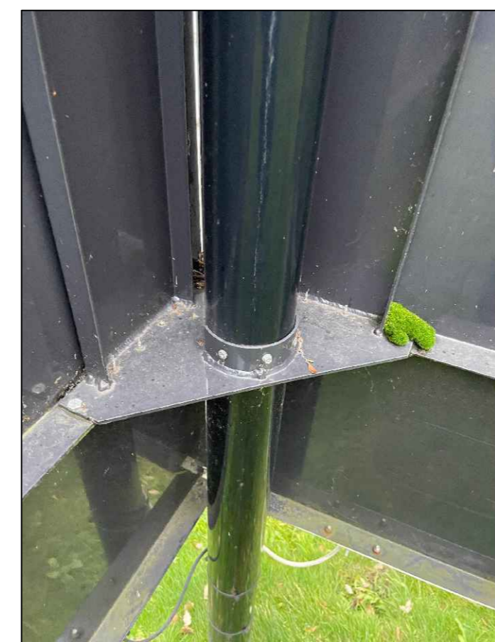
Photo of central column support bracket
