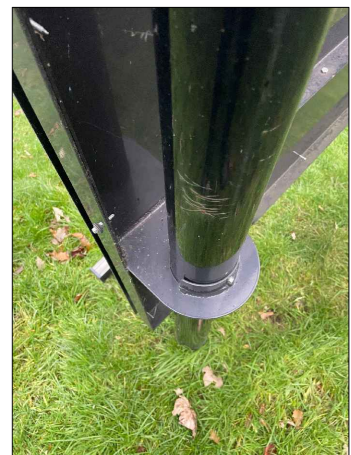
Photo of end column support bracket
