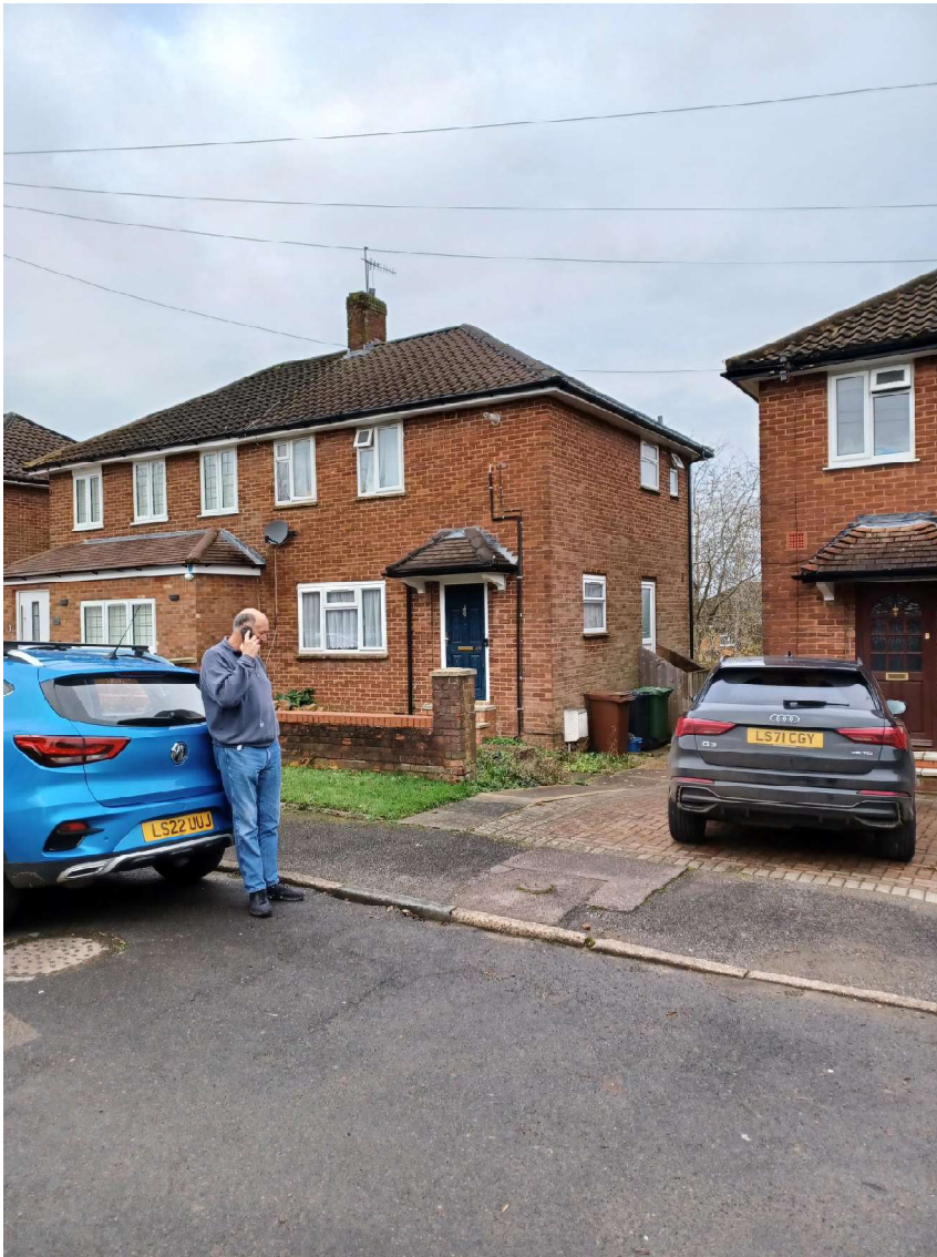
Part front elevation (right hand side) and the adjacent property 49 Langmead
