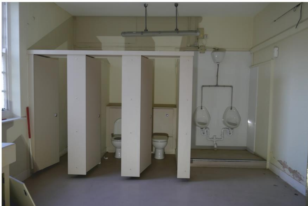
Pl. 44 Modern cubicles and sanitary ware, looking east. A hardboard panel above the cubicles conceals the two small windows visible on the external wall.
