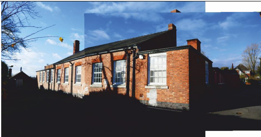
Pl. 27 South range, looking north-west
