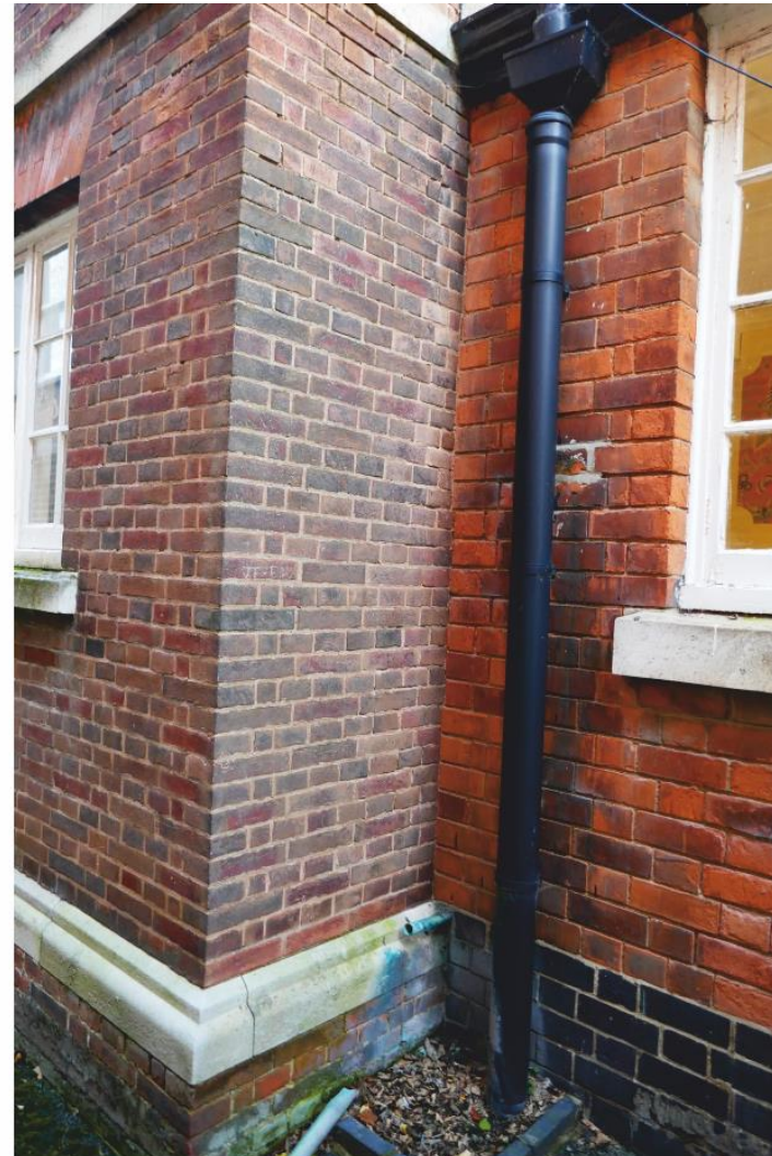
Pl. 14 Junction of front and side wings showing use of different brickwork
