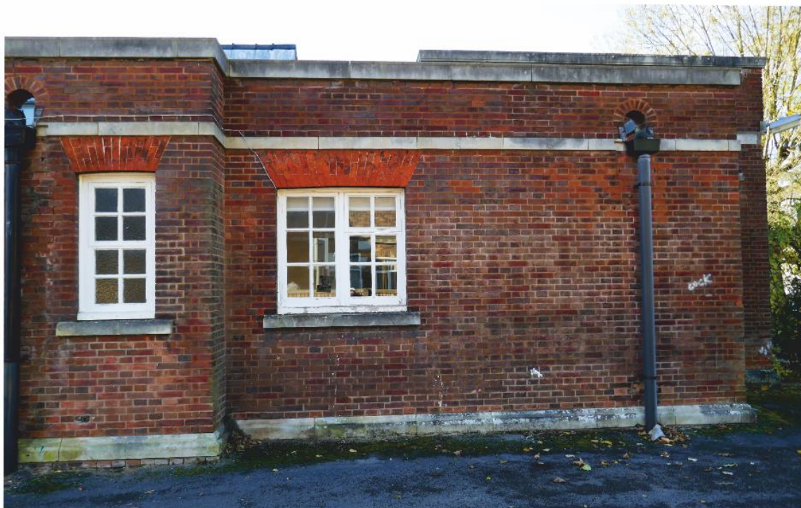
Pl.20 East elevation showing red tapered lintel bricks above the windows
