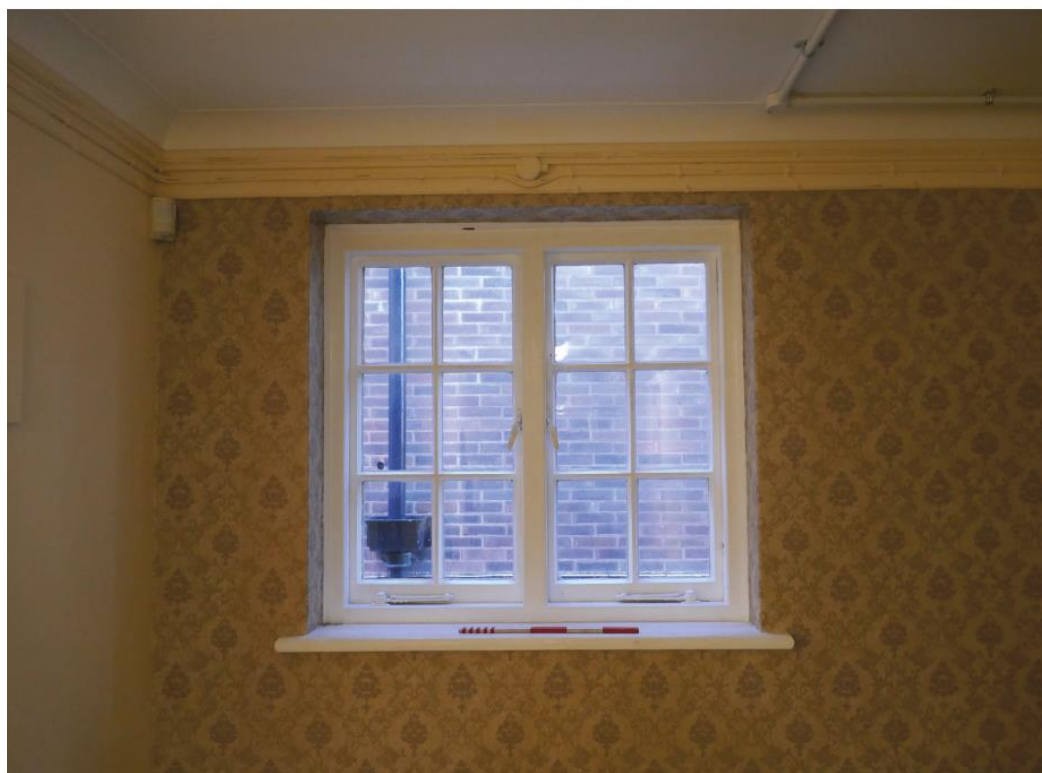
Pl. 32 Casement window at west end of corridor
