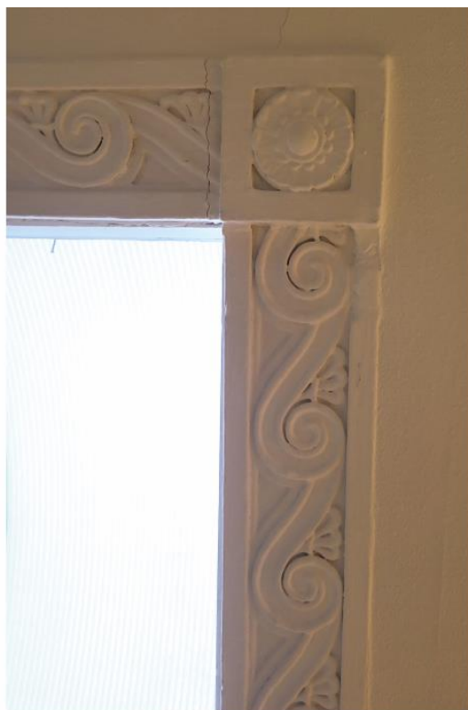
Pl. 31 Detail of moulded plasterwork around the corridor ceiling lights
