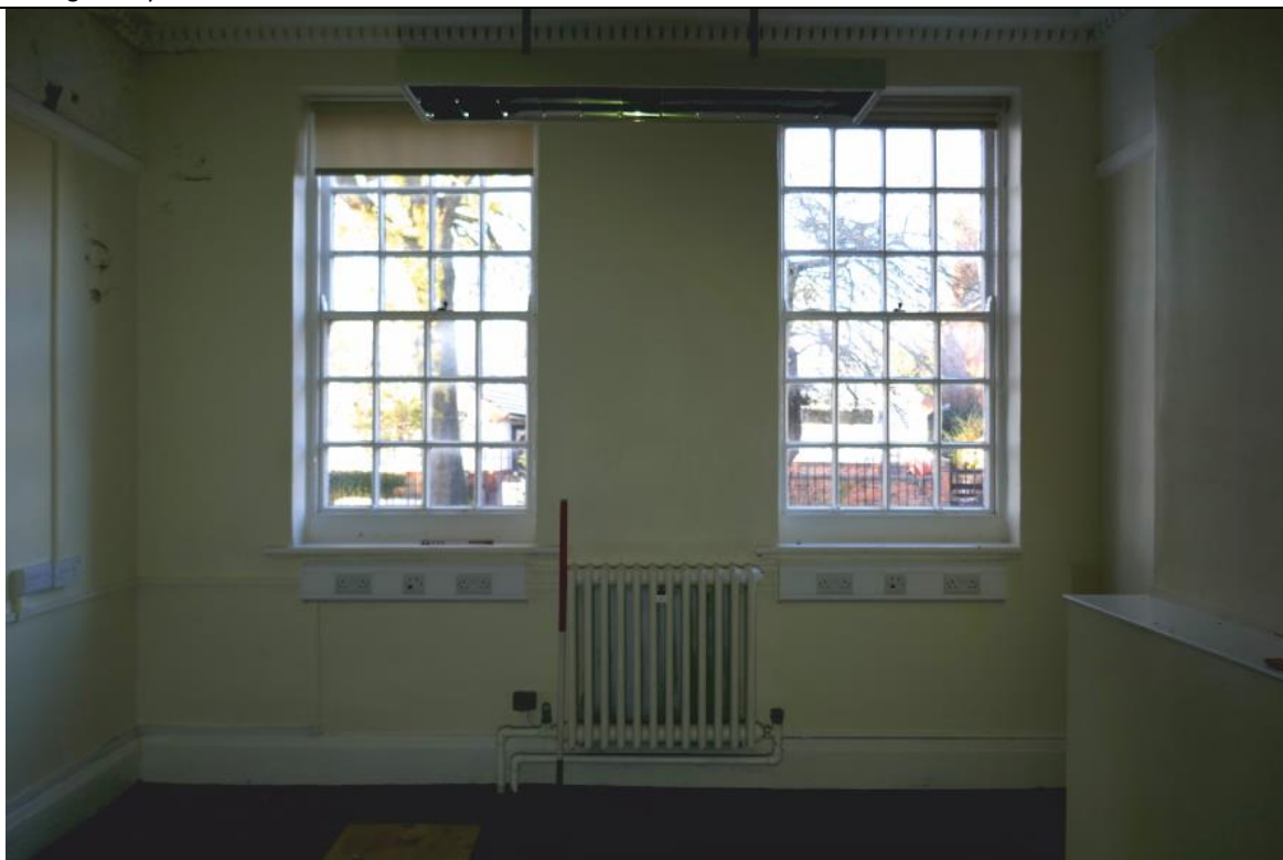
Pl. 49 Windows overlooking the front , with early radiator between.
