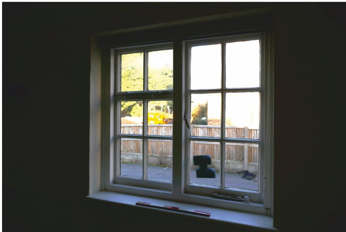
Pl. 38 Office 2 window in east wall with original fittings
