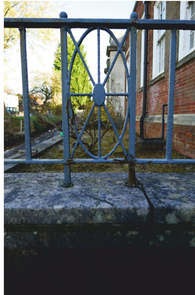
Pl. 18 Decorative oval panel with radiating spokes in metal railings at front of building
