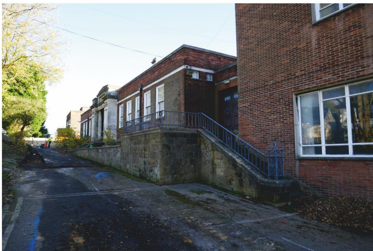
Pl. 2 College of Art building built 1930 showing the front range, looking south-east.
