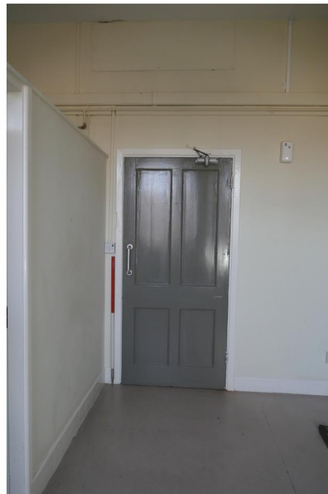
Pl. 62, Door into Ladies' toilets 9, looking south Shower and disabled toilet cubicle to left. .
