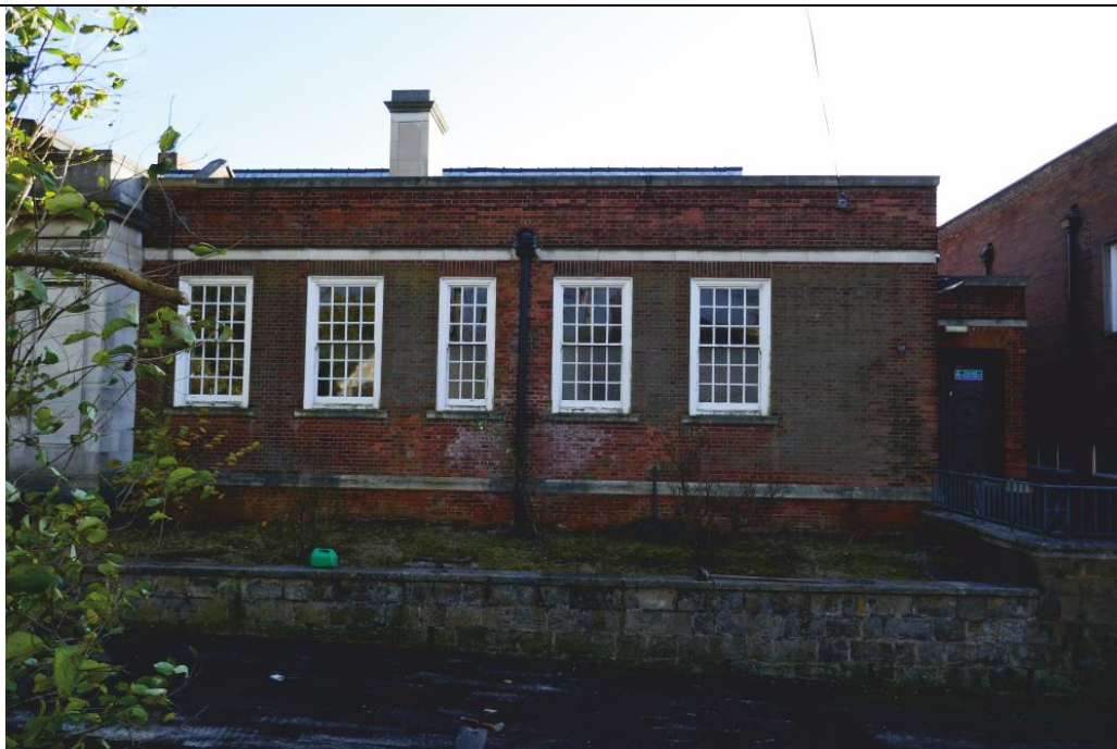
Pl.3 West part of the front range looking south
