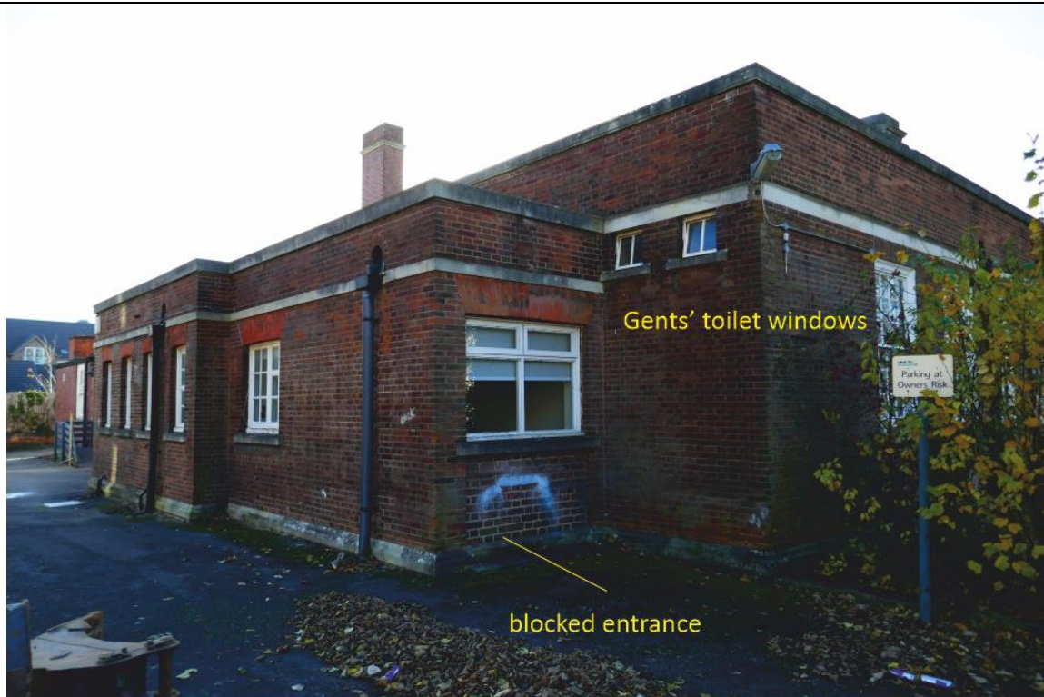
Pl.19 East elevation showing recessed wing with blocked door, looking south-west
