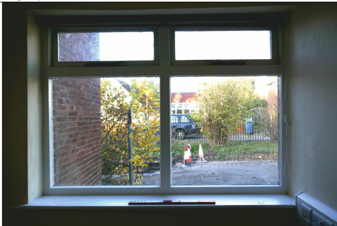
Pl. 37 Office 2 inserted window with top opening lights, looking north
