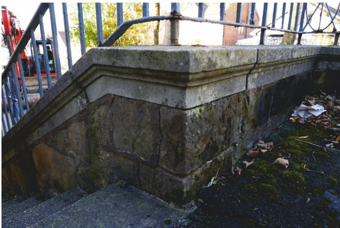
Pl.16 Detail of stone wall capping
