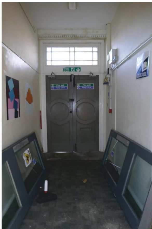
Pl. 53 Central door looking north, showing dentil coving above the fanlight.
