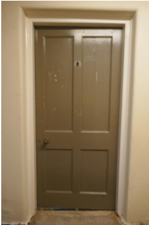
Pl. 41 Original four-panelled door into Gents' toilets
