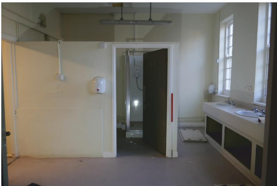
Pl. 46 Inserted shower and cubicle, looking west.
