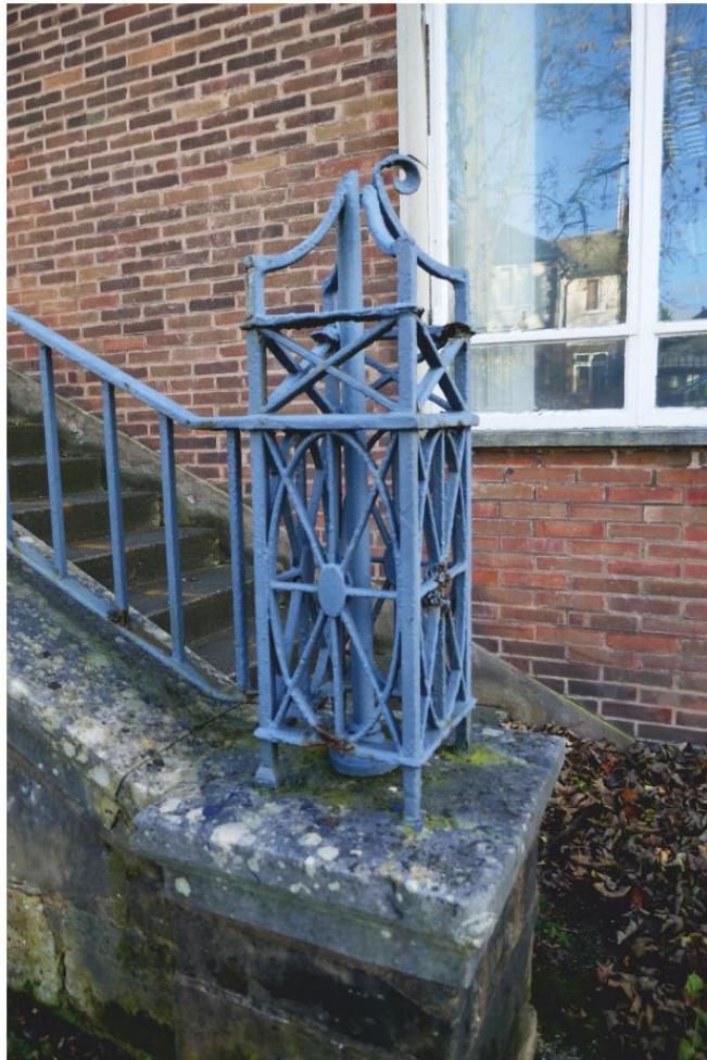
Pl. 17 Decorative 'newel' on stair at west end of the building
