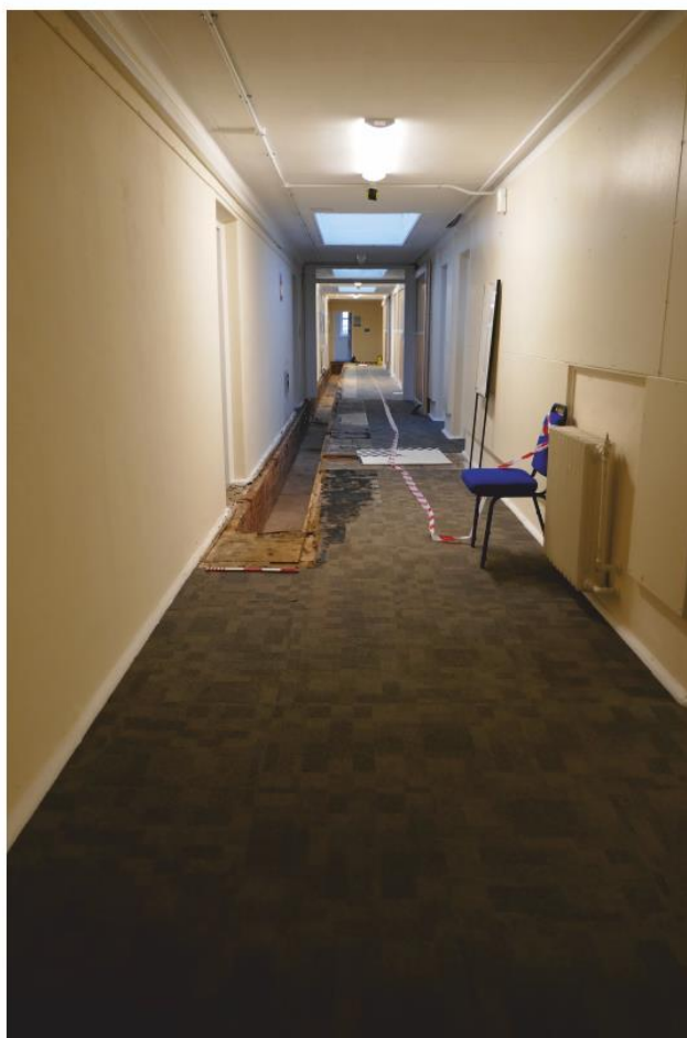
Pl. 28 North corridor, looking east
