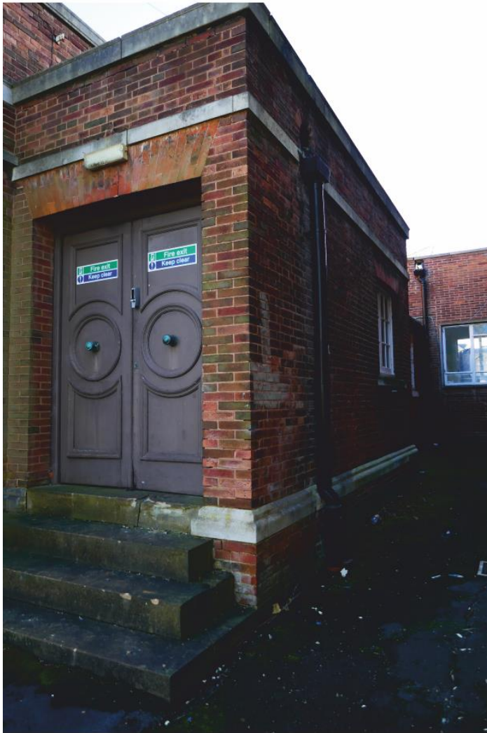
Pl. 13 West Entrance showing later link building to rear, looking south
