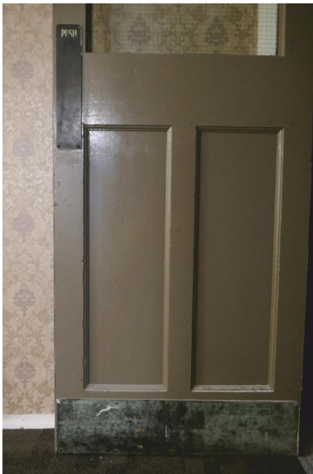
Pl. 67 Swing door showing scuff plate and finger plate
