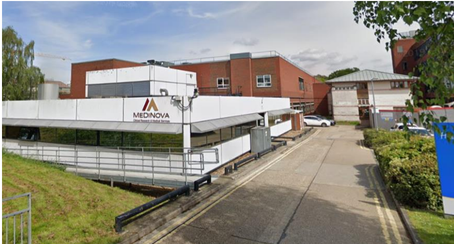
Figure 4.2 Former Medinova building
