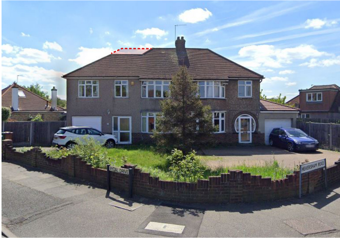
Street view from Rydal Drive showing the proposed change to the existing roof profile, highlighted in red.
