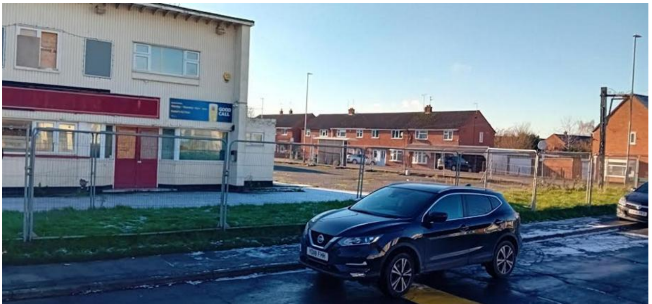
Photo D - View of Former Nautical William PH from north-east towards Rolleston Road
