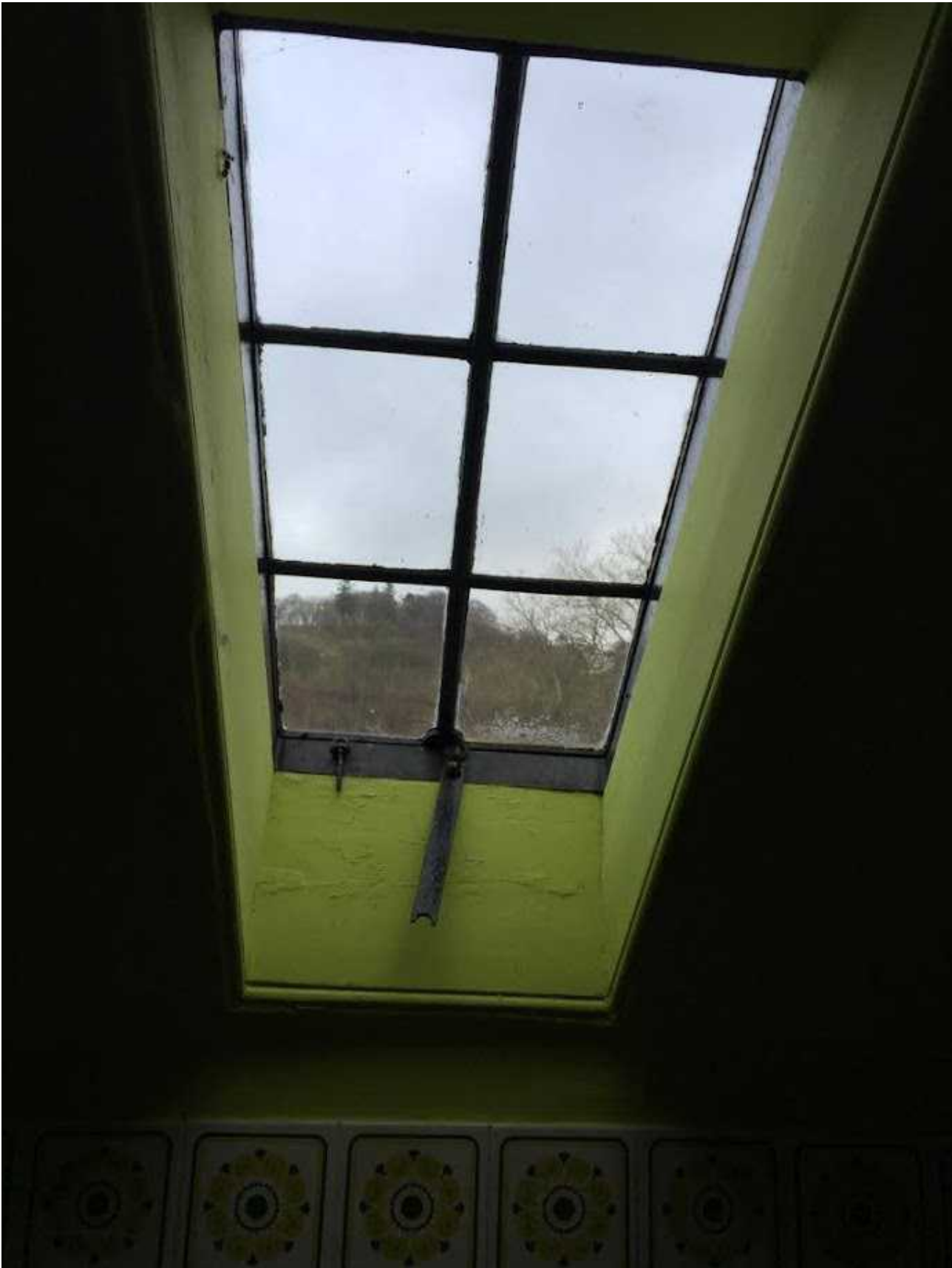
Existing metal roof lights
