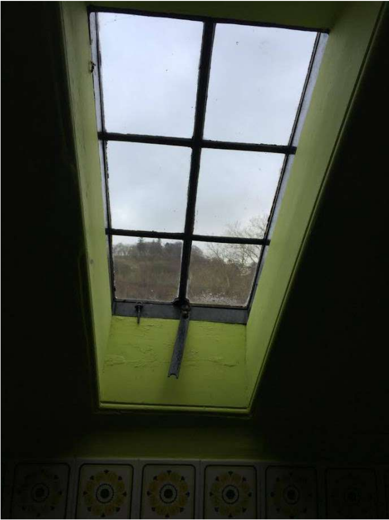
Existing metal roof lights
