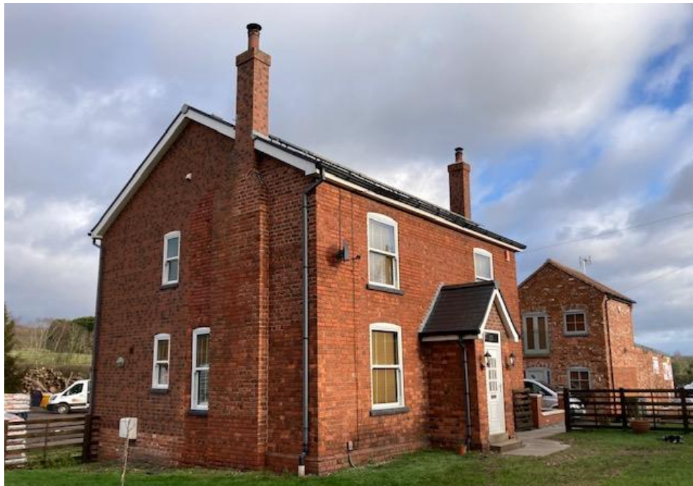
10. The south west corner of the house.
