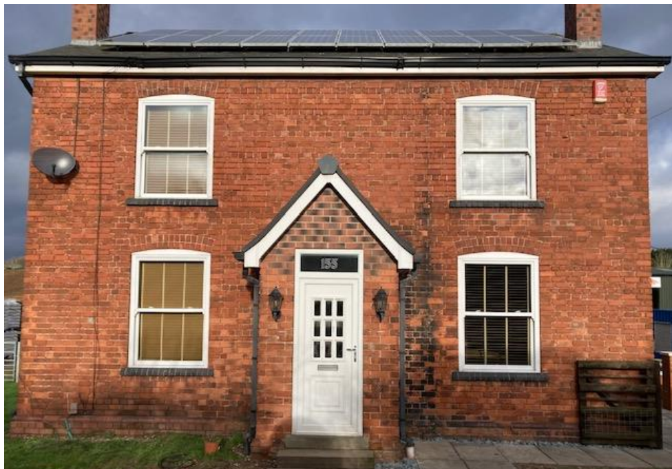
11. The front south elevation.
