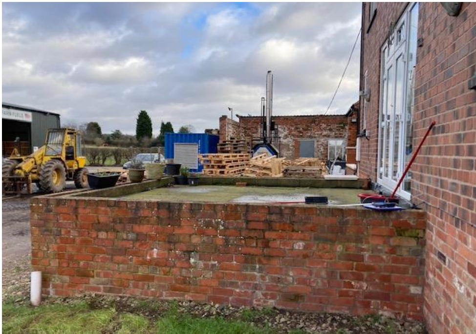
8. Looking west across the rear extension base.
