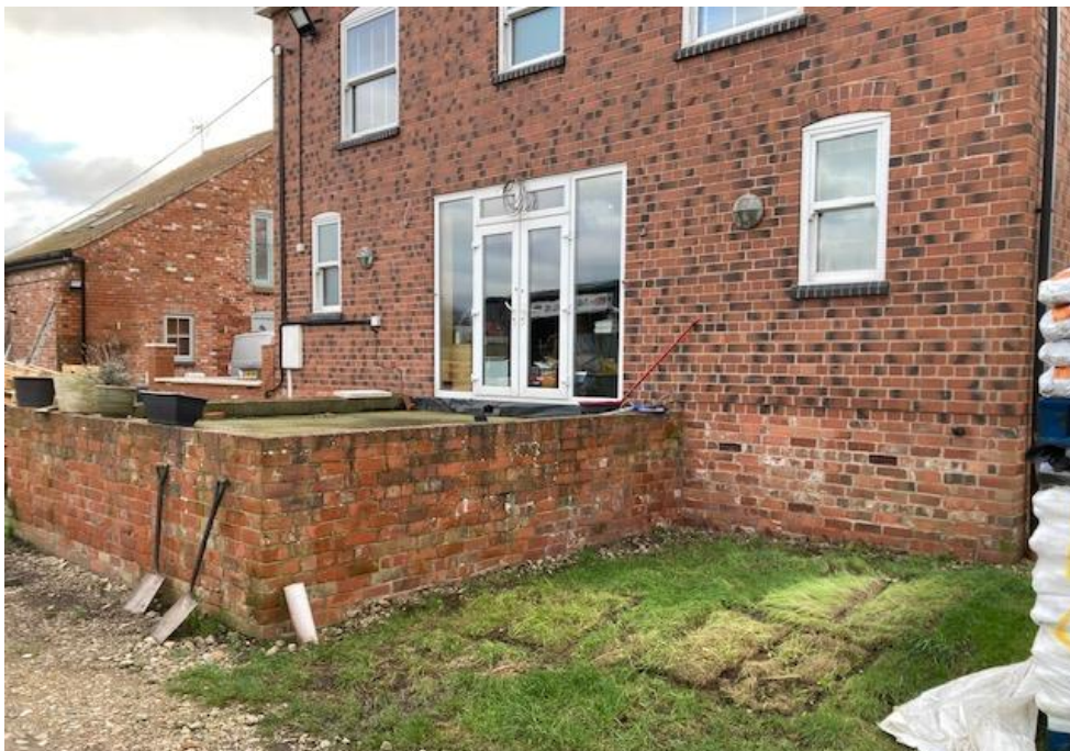
7. The north west side of the rear extension base.
