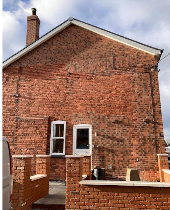
2. The east gable end of the house.
