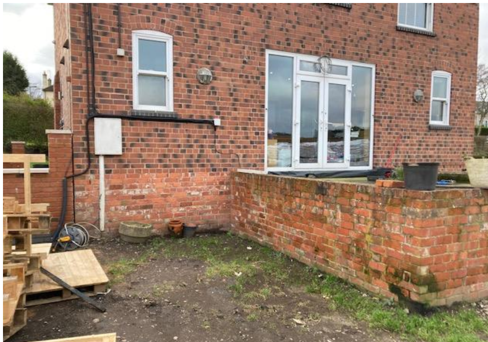
5. The base of a proposed extension (not completed) –north east side.
