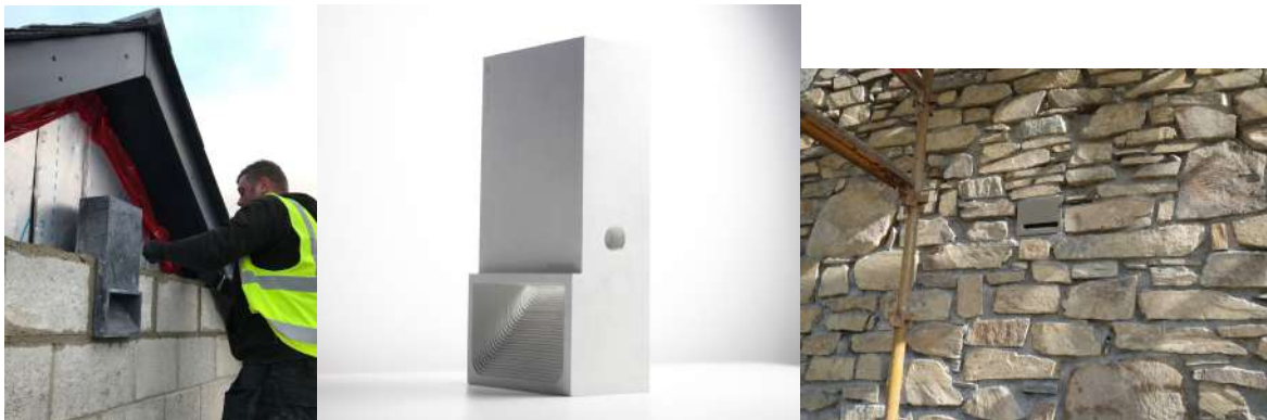
Photograph 7. Green and Blue' bat block and woodstone bat box `
