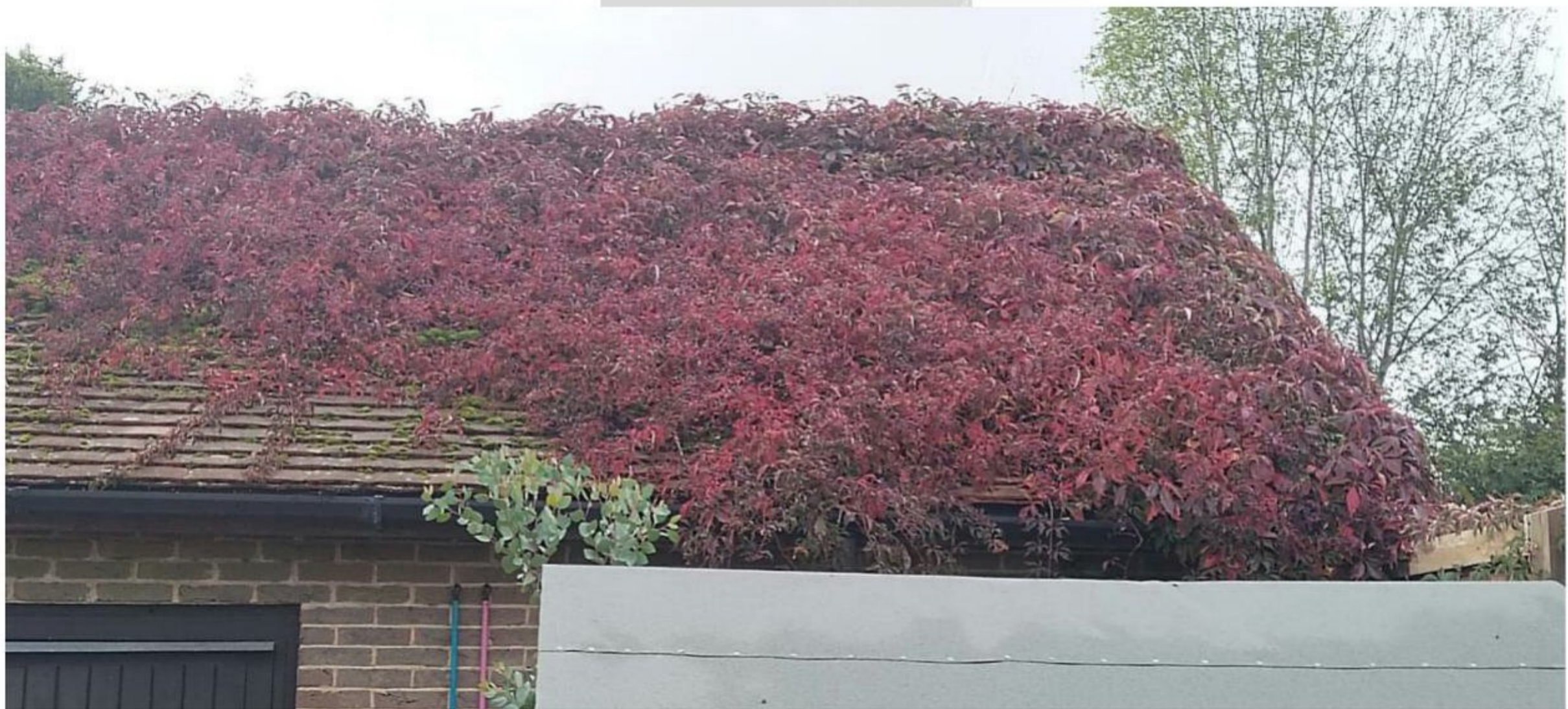
Photograph 6: Virginia creeper on garage that precludes bat access
