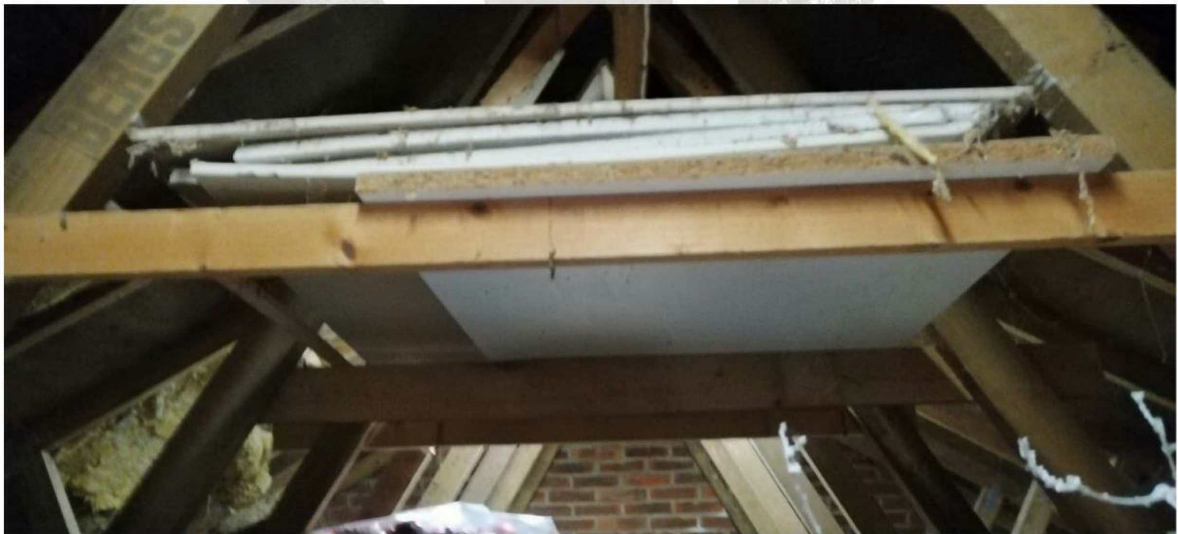
Photograph 5: Garage roof void
