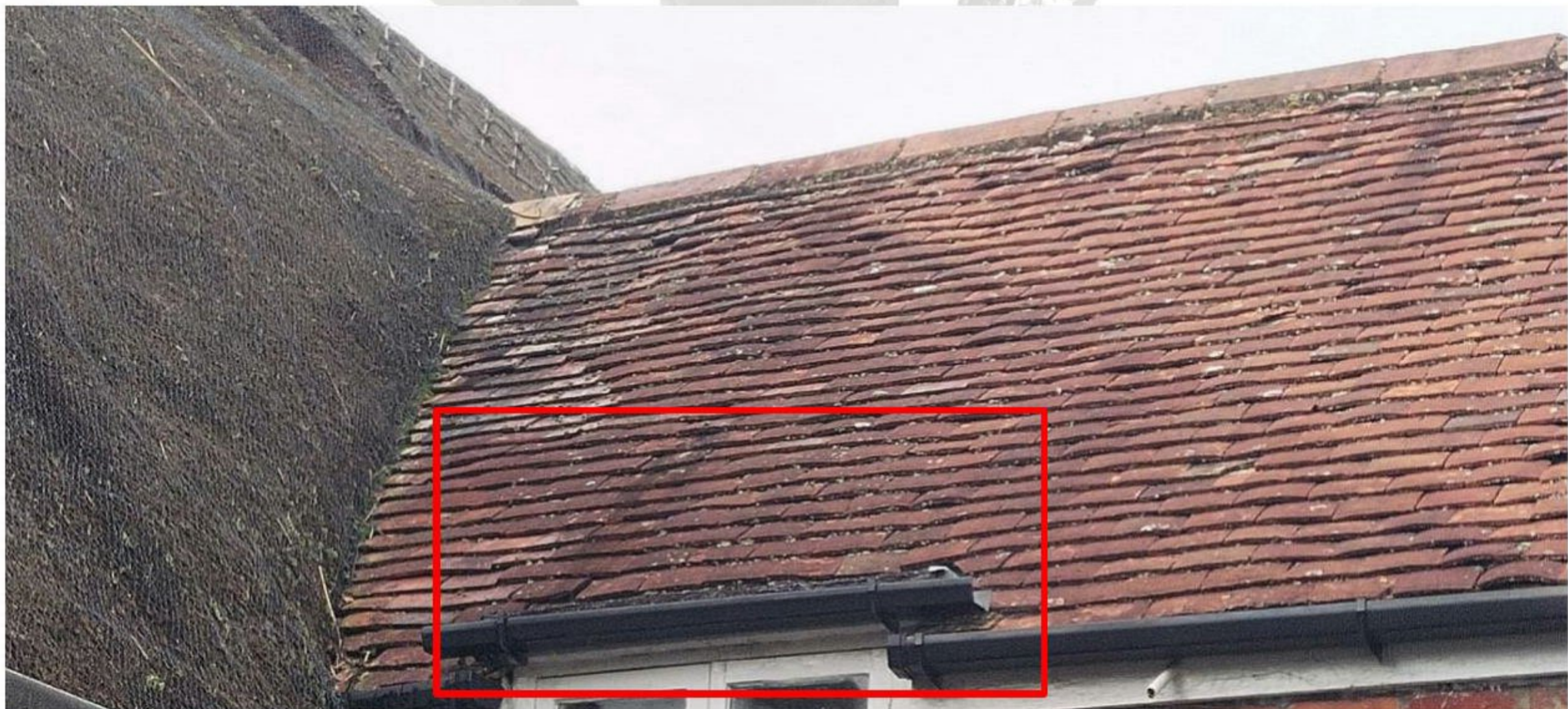
Photograph 2: Tightly fitted roof tiles in location of proposed door
