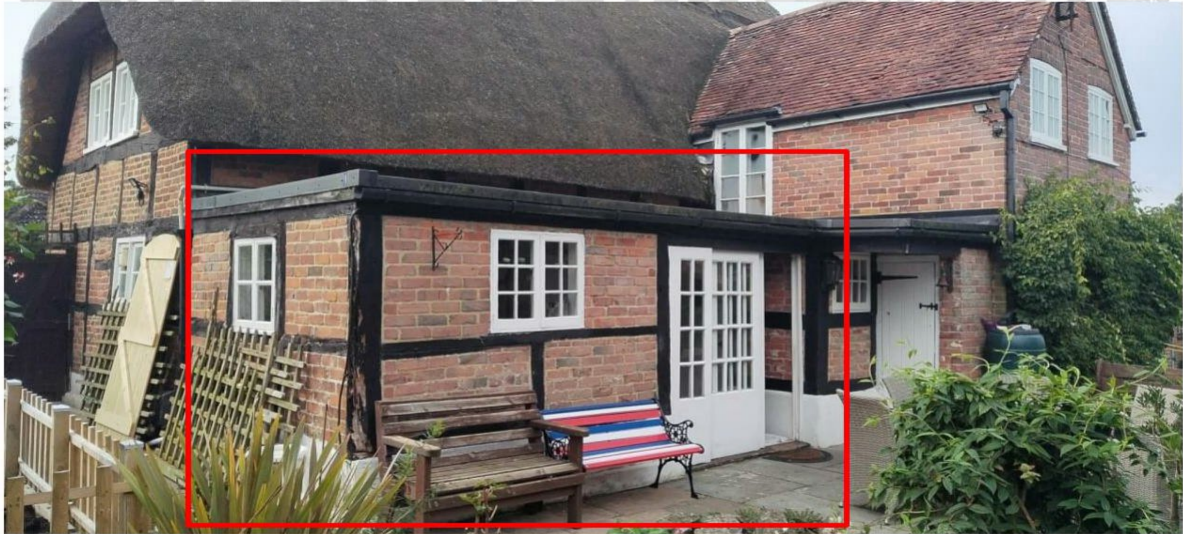
Photograph 1: Flat roofed extension scheduled for demolition & rebuild
