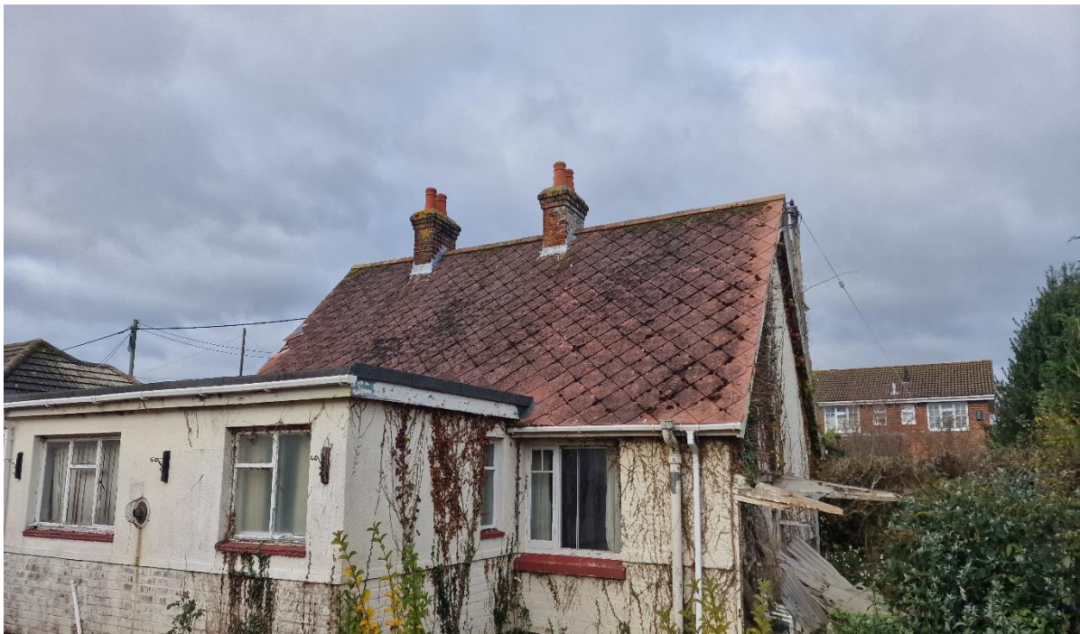
Picture 2: Showing the rear elevation.
