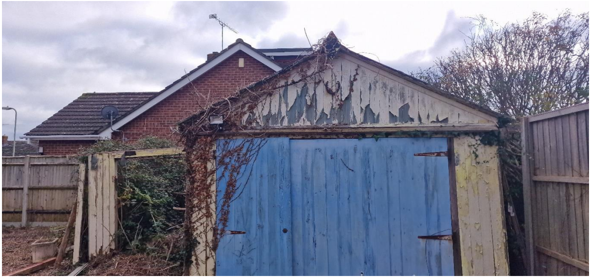
Picture 3: The front of the garage structure.
