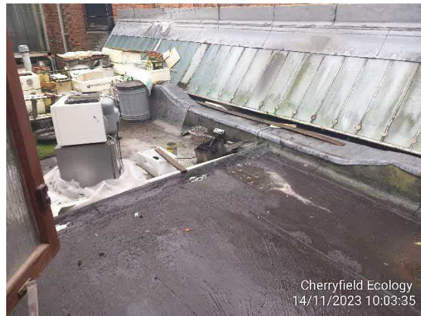
Figure 3: Flat bitumen felt extension to the rear of B1
