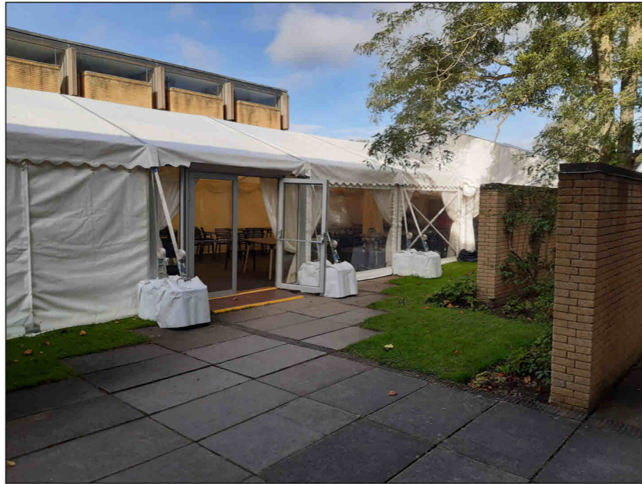
View 8 Looking north-west to marquee with Dining Hall behind
