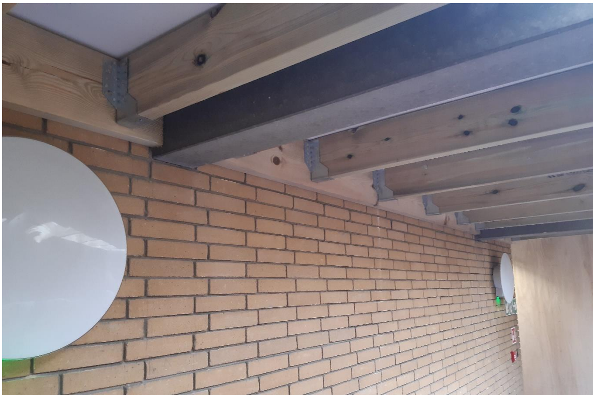
Temporary timber joists and wall plates installed in a staircase
