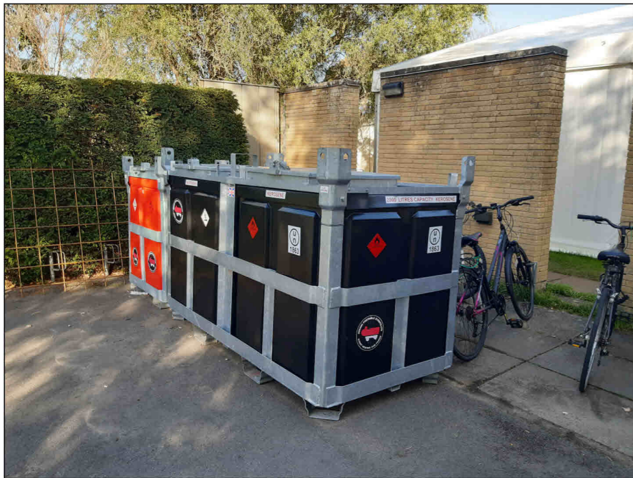
View 4 Looking at fuel store
