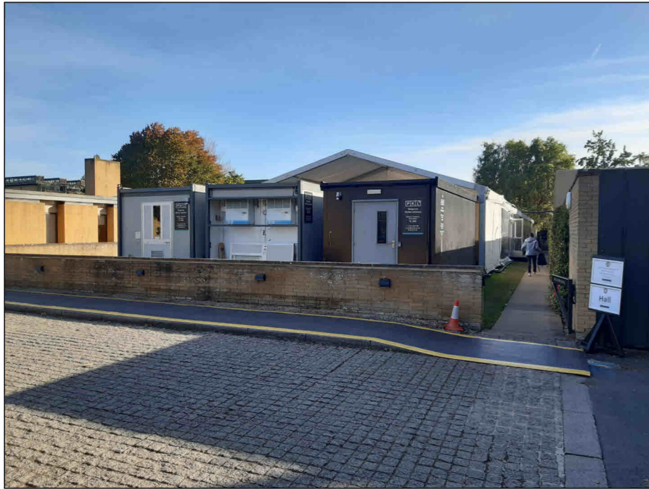
View 1 Looking south-east from main entrance area to temporary kitchen
