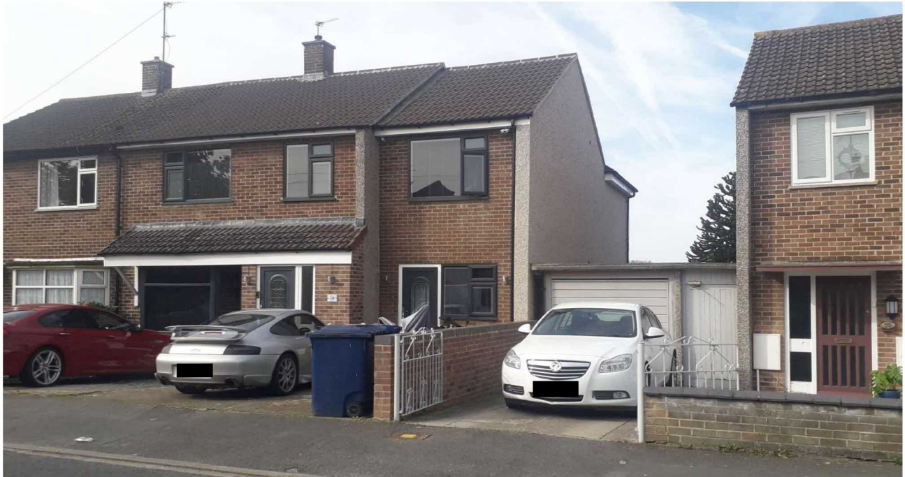
Existing gap between N°22 & N°24a
