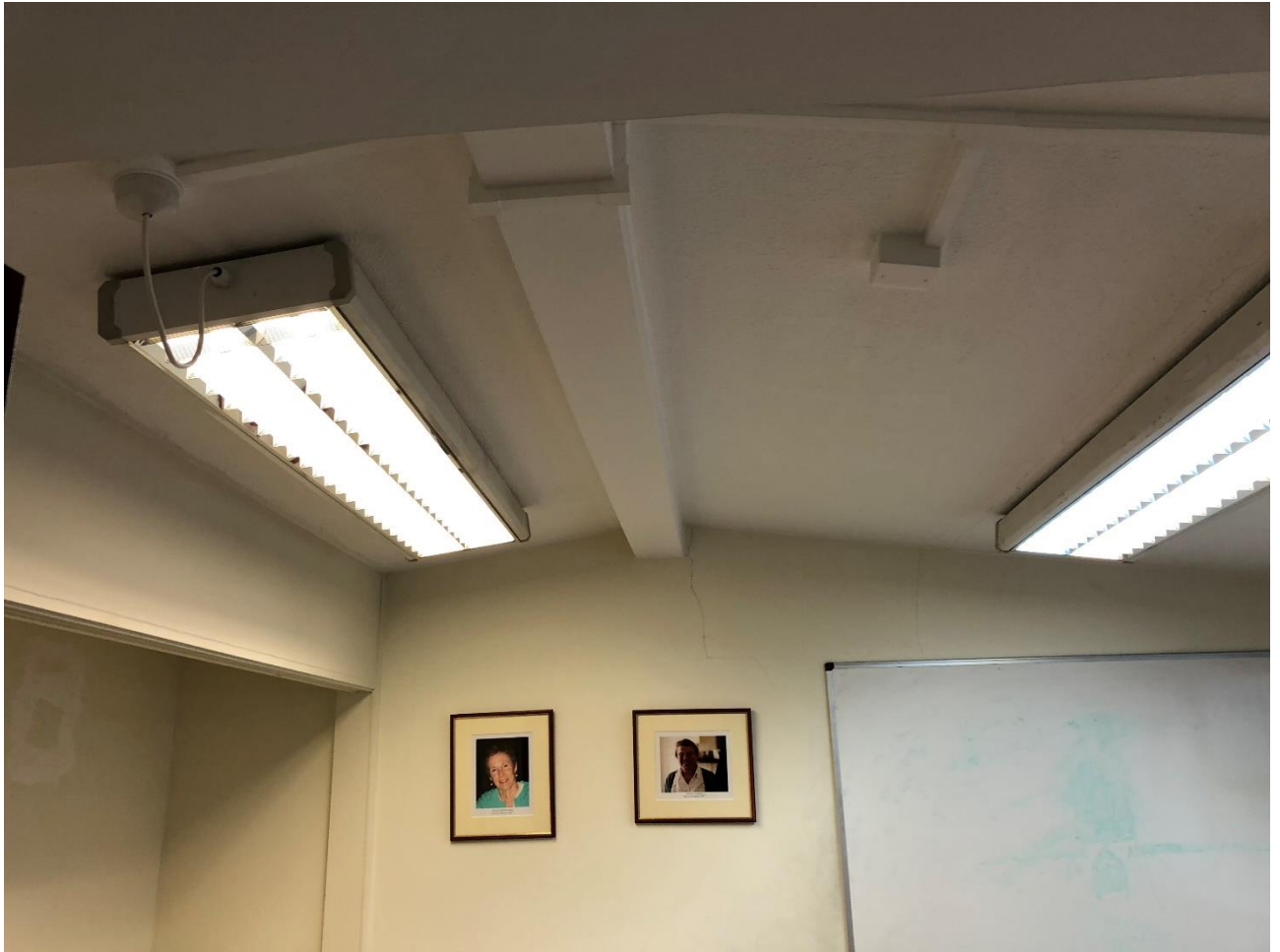
Photograph 10- Cracking in Gable Wall Computer Suite
