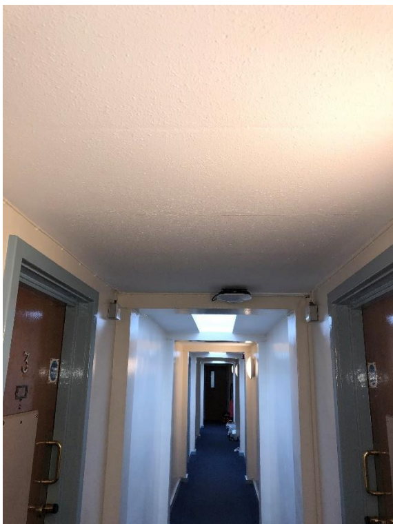
Photograph 3- RAAC Corridor Bay
