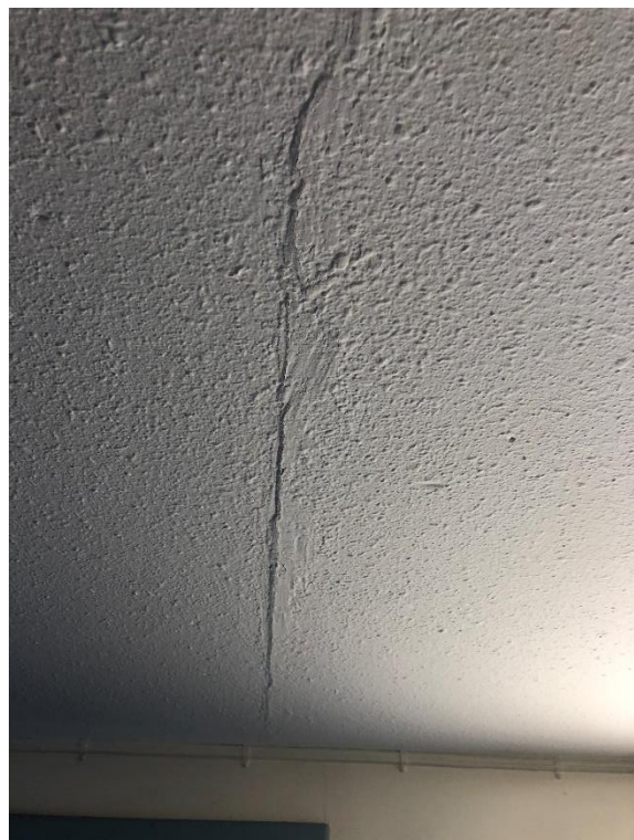
Photograph 4- Typical Joint Between RAAC Corridor Panels
