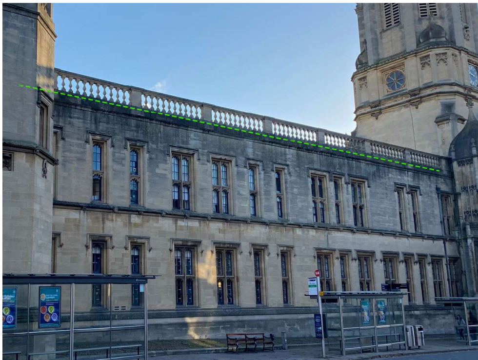
Fig 19: Photomontage of proposed photovoltaic installation (Not visible from this viewpoint). The position is indicated with the dashed green line.
