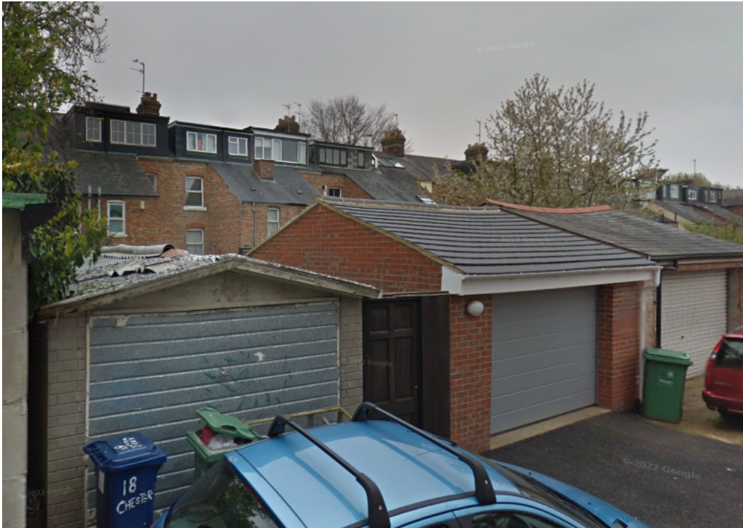
Existing Garage (lhs) facing the lane to the rear
