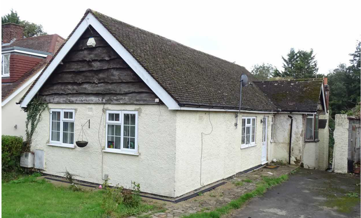
Image 1 – South & West facing elevation of the property
