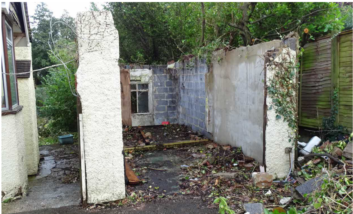
Image 8 – Detached garage located to the South of the main dwelling
