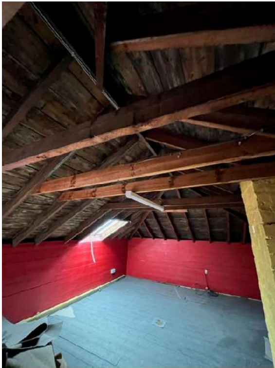
^ Existing attic as existing
