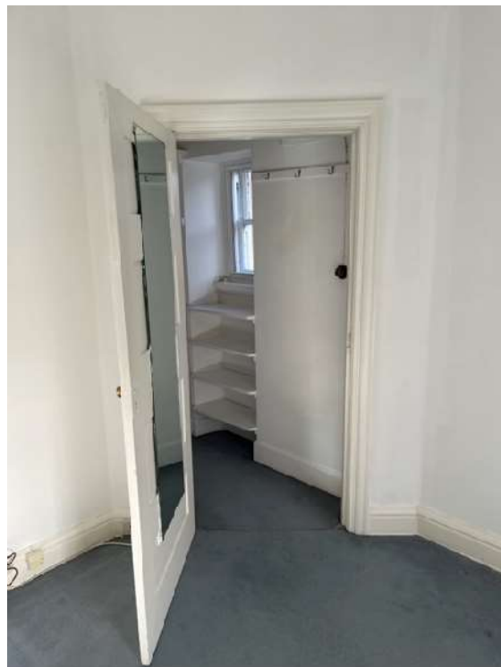
^ Existing door and cupboard within bedroom
