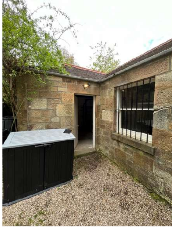
^ Garage pedestrian door as existing
