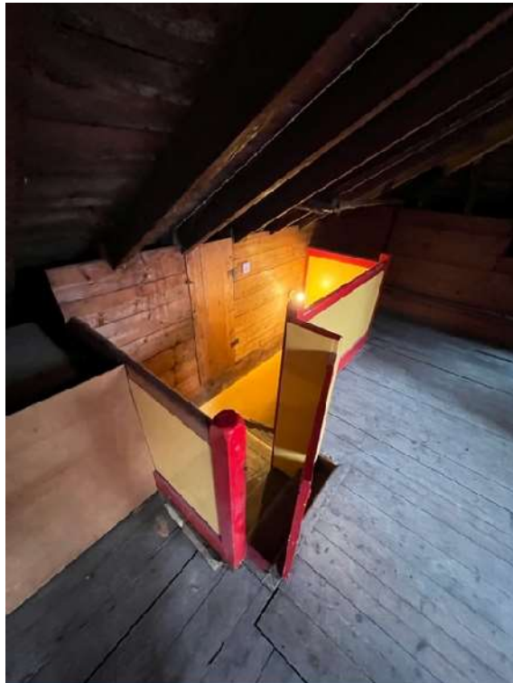
^ Existing access from bathroom to attic
