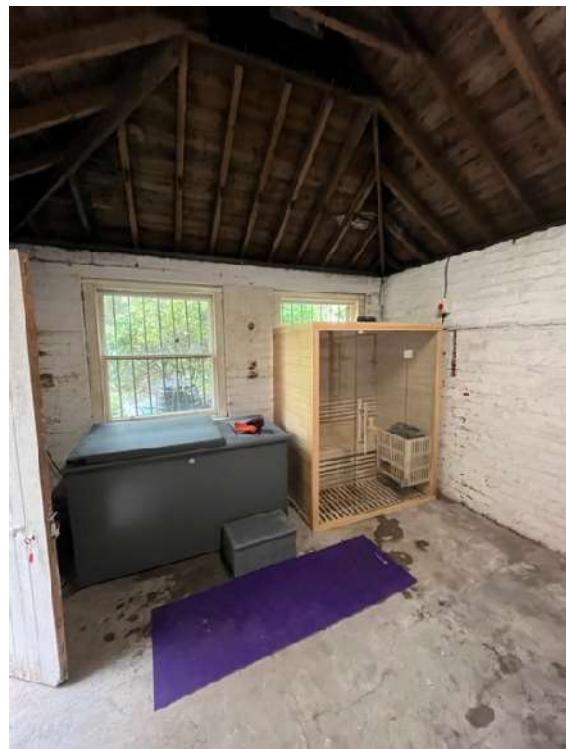
^ Existing garage internals as existing
