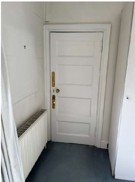
^ Existing door from bedroom to bathroom
