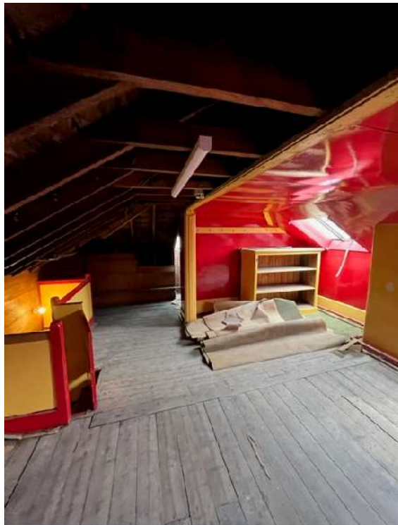
^ Existing attic as existing
