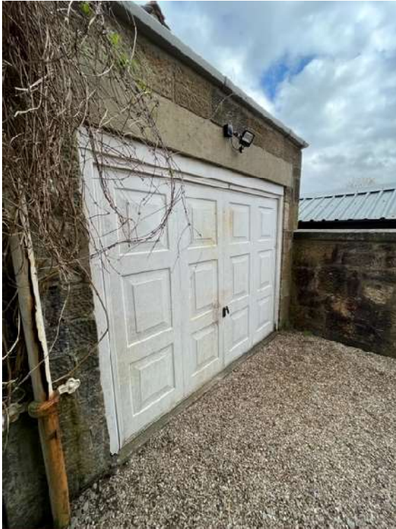
^ Garage door as existing
