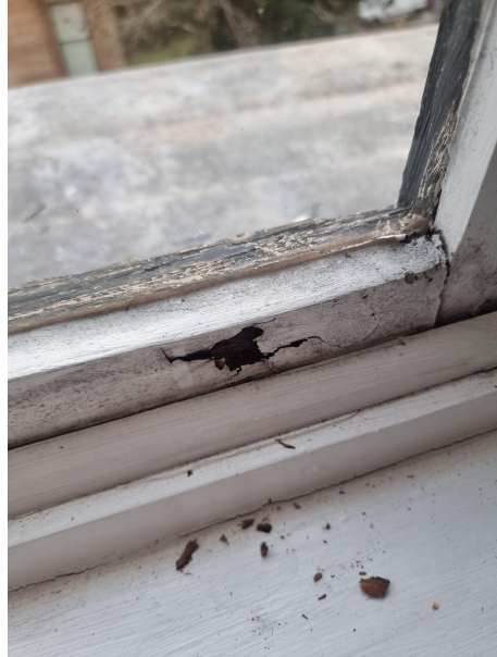
The internal sill to the arched window is rotting due to water ingress. The second photo shows the water damaged and rotting bottom rail. There is also a large seal which has been put in place temporarily to stop the wind and water entering.
