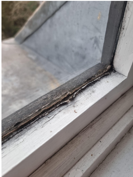
The first photo shows the seals to the glass are coming away and failing. The second photo again shows the large seal which has been installed as a temporary fix. It also shows that the window is becoming unattached at the joints.
