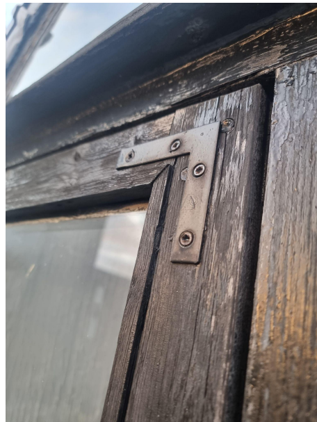
The astragal to the window is badly weathered and damaged. The second photos shows that the joint are currently being held together with brackets as the existing screws are unable to keep it securely together.
