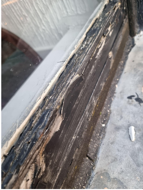
The bottom rail is severely water damaged and rotting externally and the mastic is broken in areas.
