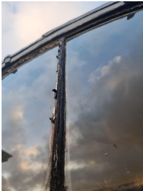
The astragal to the window is badly weathered and damaged. The second photos shows that the joint are currently being held together with brackets as the existing screws are unable to keep it securely together.
