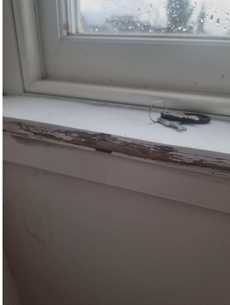
The internal sill to the arched window is rotting due to water ingress. The second photo shows the water damaged and rotting bottom rail. There is also a large seal which has been put in place temporarily to stop the wind and water entering.
