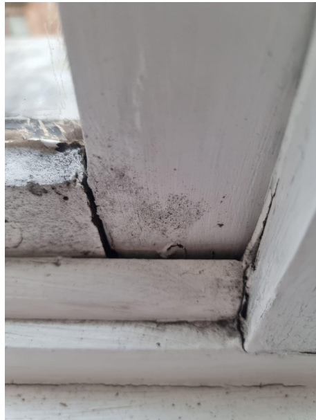
The first photo shows the seals to the glass are coming away and failing. The second photo again shows the large seal which has been installed as a temporary fix. It also shows that the window is becoming unattached at the joints.
