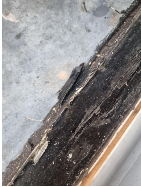
The bottom rail is severely water damaged and rotting externally and the mastic is broken in areas.
