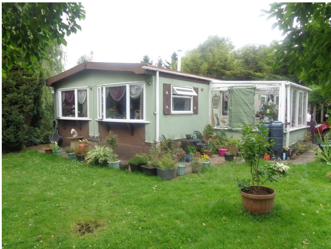
PHOTO 1 – STOREY LODGE FROM SOUTH-EAST
