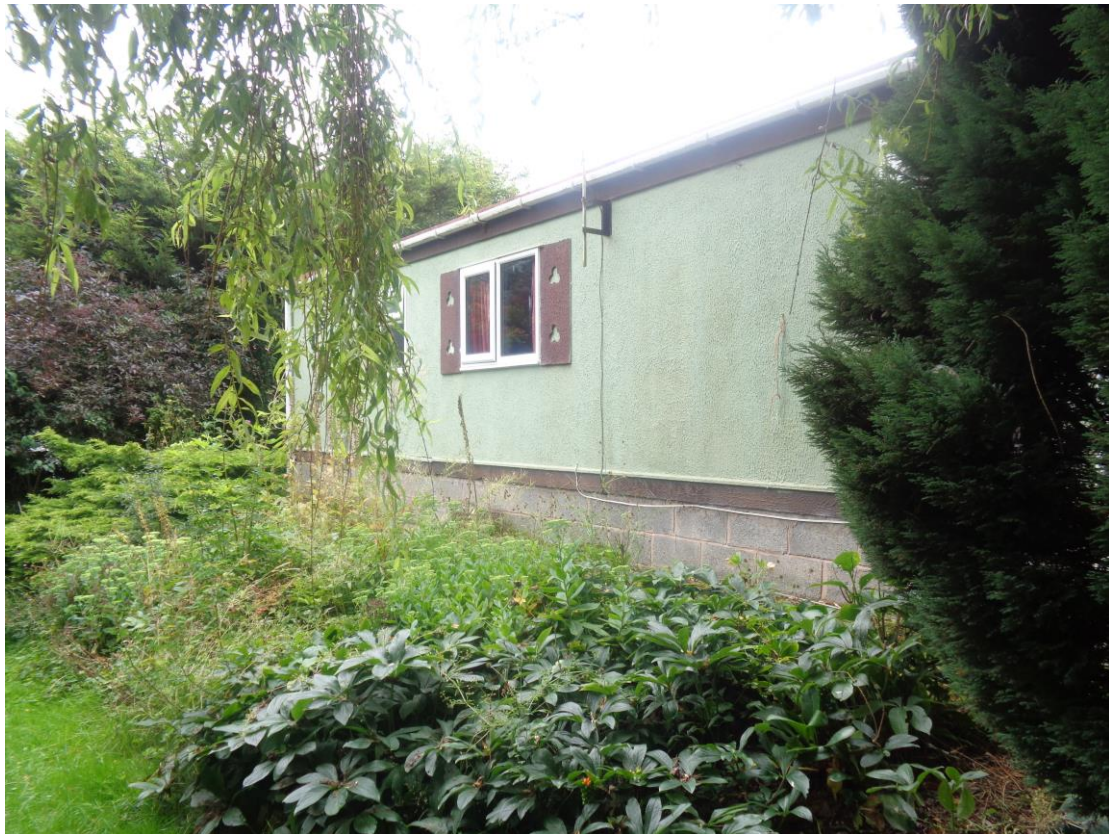
PHOTO 2 – STOREY LODGE FROM WEST SIDE
