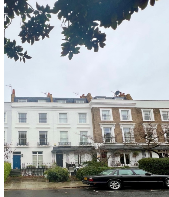
45 Northumberland Place, the building
