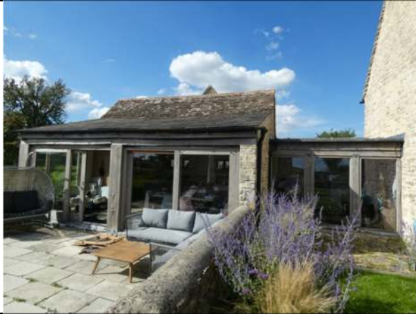
Photograph 1. The south elevation of the breakfast room
