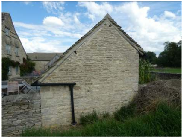
Photograph 10. The west elevations of the garden store
