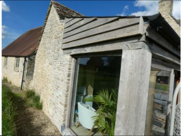
Photograph 2. The west elevation of the breakfast room
