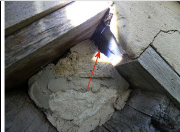
Photograph 13. Small opening at the top of the east gable wall of the garden store
