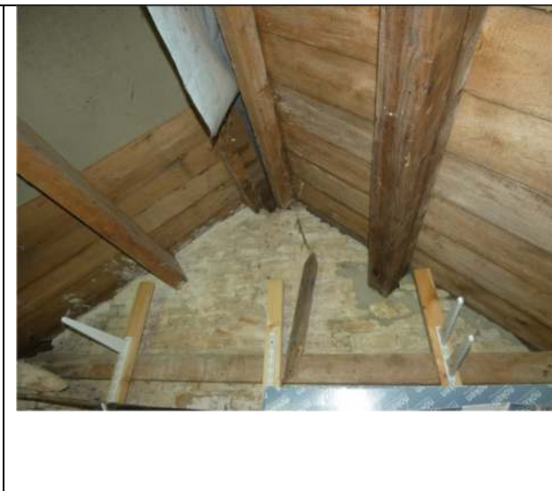
Photograph 16. Exposed timbers in the garden store
