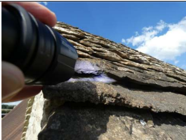
Photograph 5. Example of the slates on the roof of the kitchen
