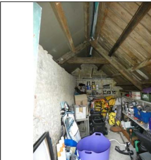
Photograph 15. The interior of the garden store
