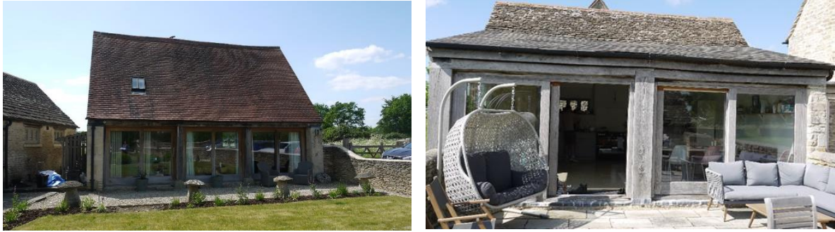
Plate 3 (left) Curtilage listed cart shed to the northwest of the farmhouse now annex and plate 4 rear addition to remodded piggery attached to farmhouse.
