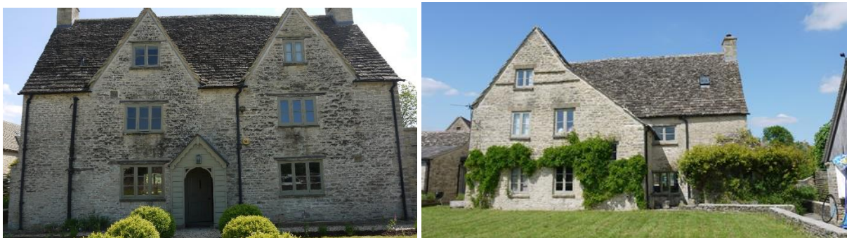
Plate 1 (left) Grade II listed Mill Farmhouse and Plate 2 (right) rear elevation of Mill Farmhouse.
