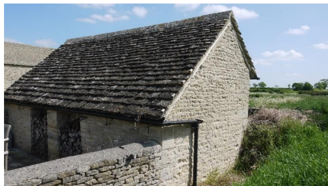
Plate 8 Existing Piggery and garden store proposed for reuse as garden room.
