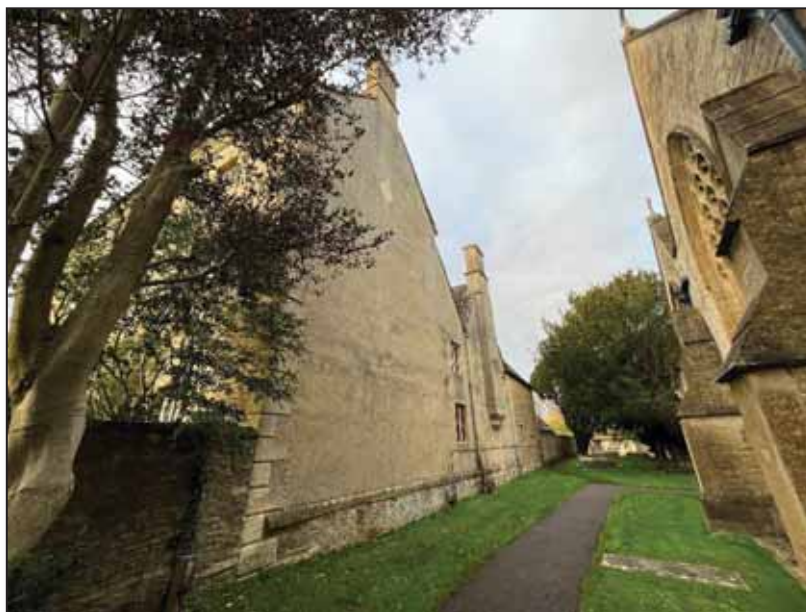
Image 15: East elevation showing low stone course above plinth
