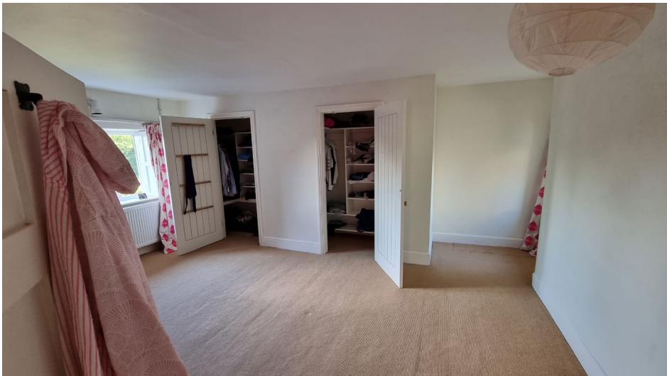
Modern joinery to be removed to form new bathroom
