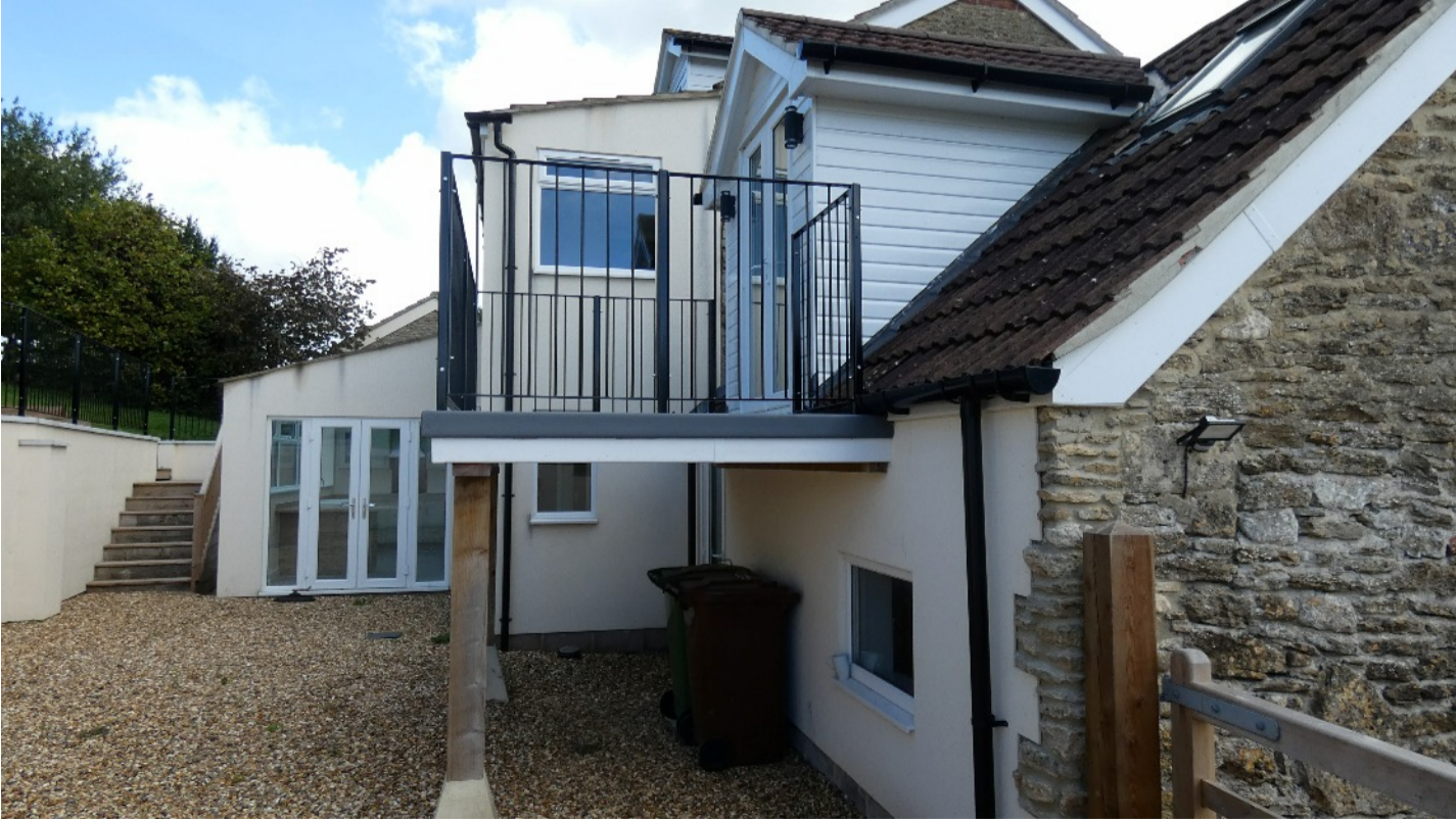
Side View from the Yard
