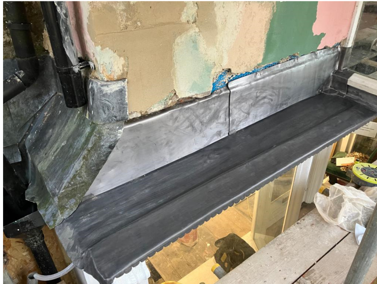
New leadwork being fitted over the shop front
