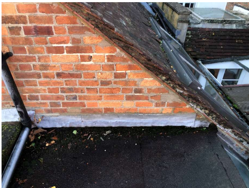
Figure 5: Utility roof junction with existing kitchen roof
