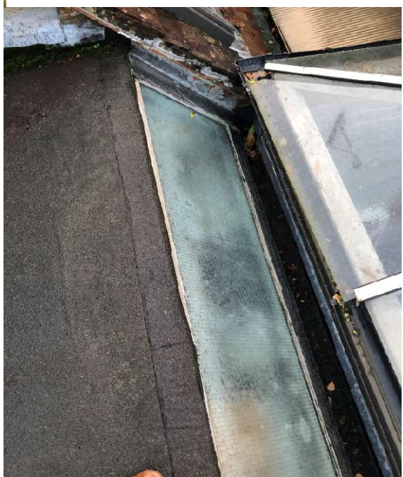
Figure 4: Existing rooflight over utility room
