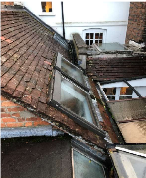
Figure 3: Roof over kitchen and existing flat roof over utility
