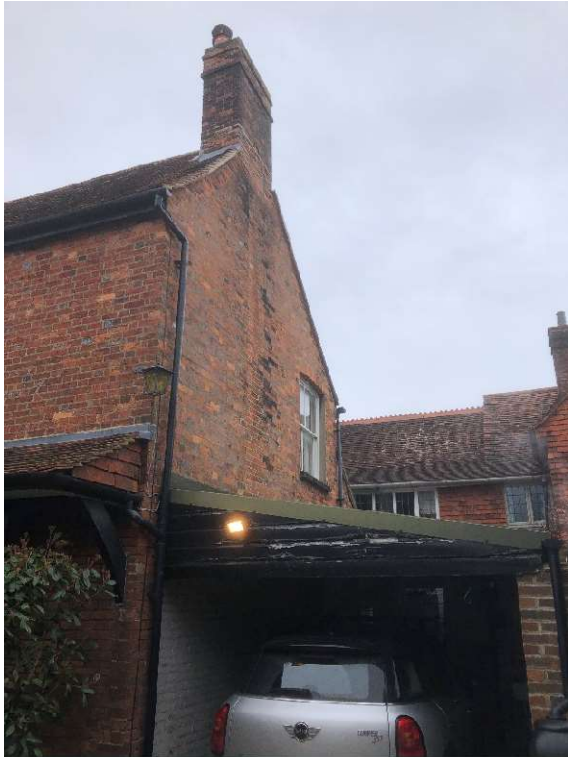
Figure 1: Existing Car port
