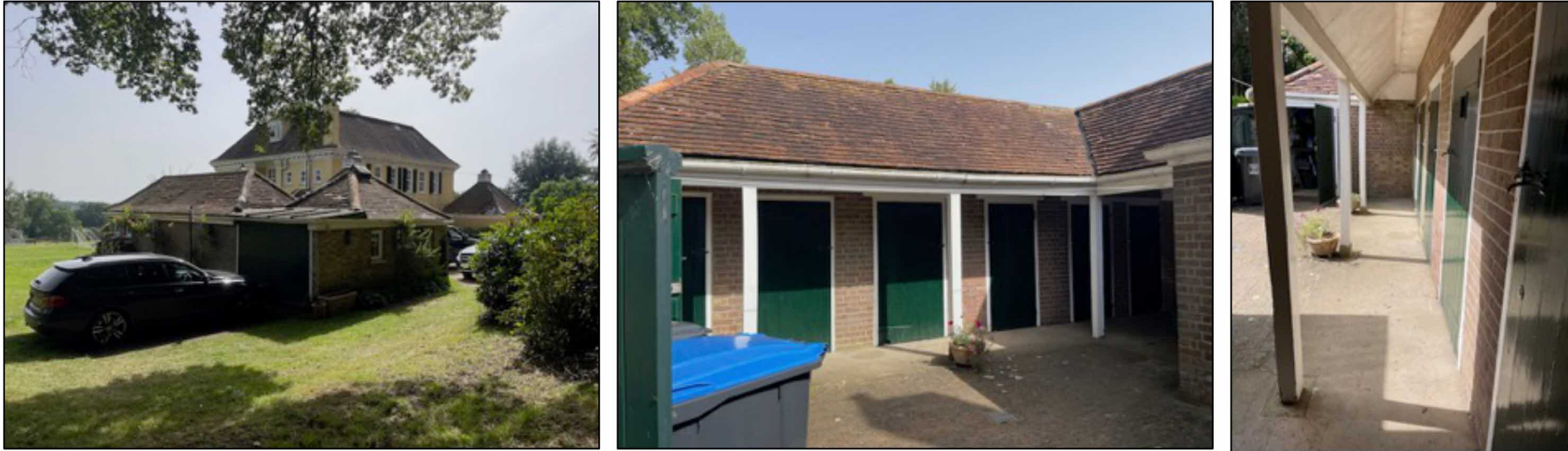
Figure 11: View of the northern courtyard of outbuildings, taken externally viewed from the west and internally viewed from the gate. Photograph © Hubbard Conservation.
