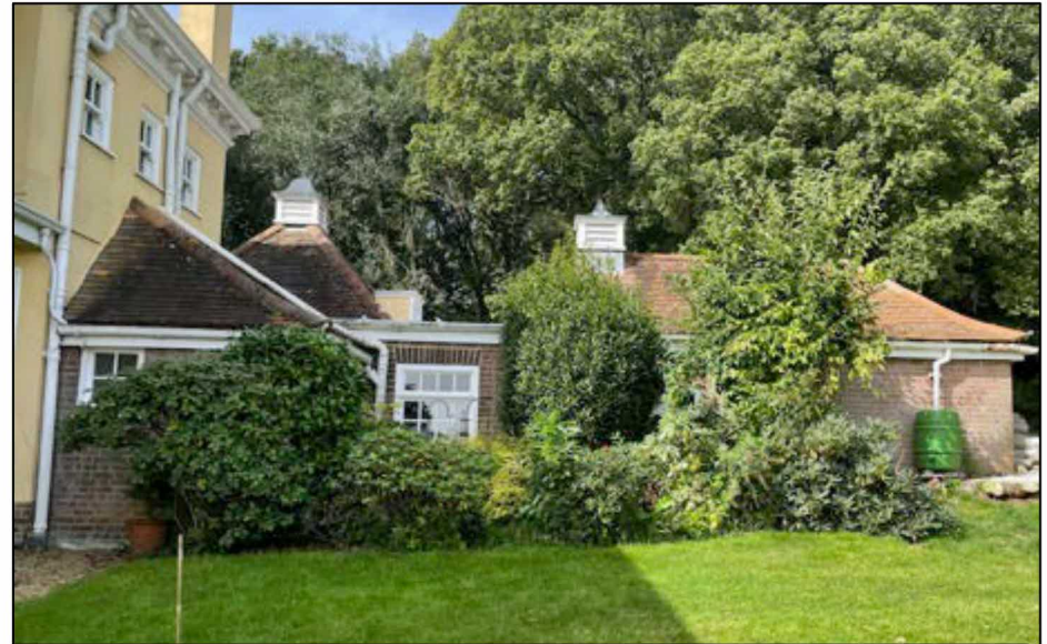
Figure 15: east side of the lean-to, flat roof extension (G1) and the outbuildings. Photograph © Hubbard Conservation.
