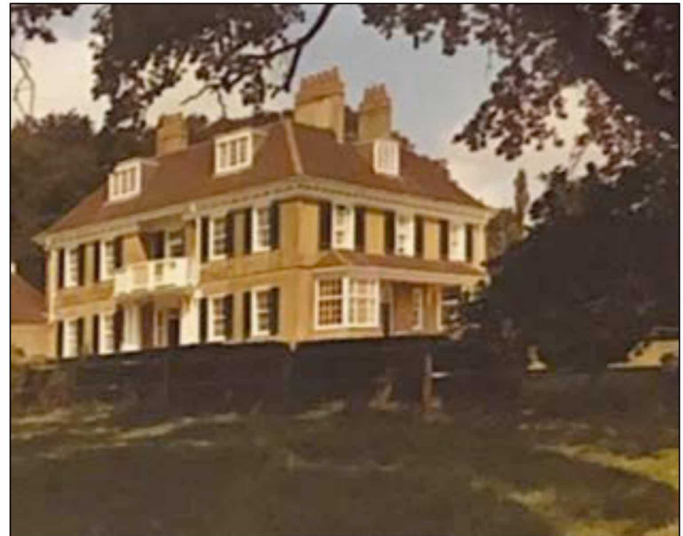
Figure 14: South and east elevation taken in the 1970s. Notice the vast chimneystacks, which were removed. Photograph © Hubbard Conservation.
