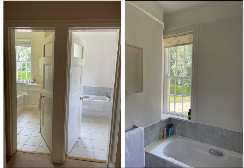
Figure 29: Rooms F1a (left) and F1b (right) the doorways of which are shown in the left hand side photograph. The right photograph shows the awkward junction of the cranked partition wall between the two bathrooms and how the wall has been created to keep the window revealed. Photograph © Hubbard Conservation.
