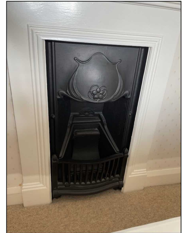
Figure 36: Fireplace in room S6. Photograph © Hubbard Conservation.
