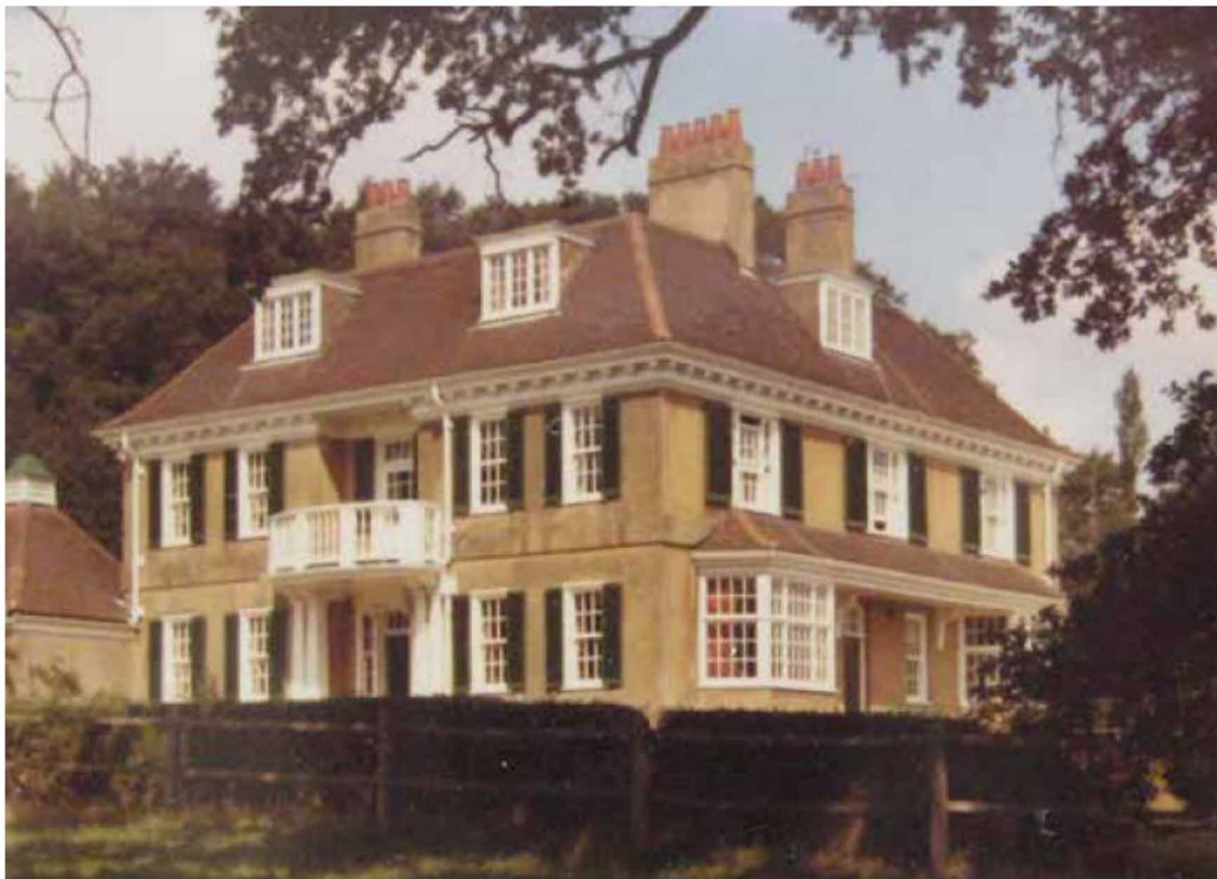
Fig.2 – Side/Rear Elevation (South-East) 1970s photograph with original chimneys shown and tired render
