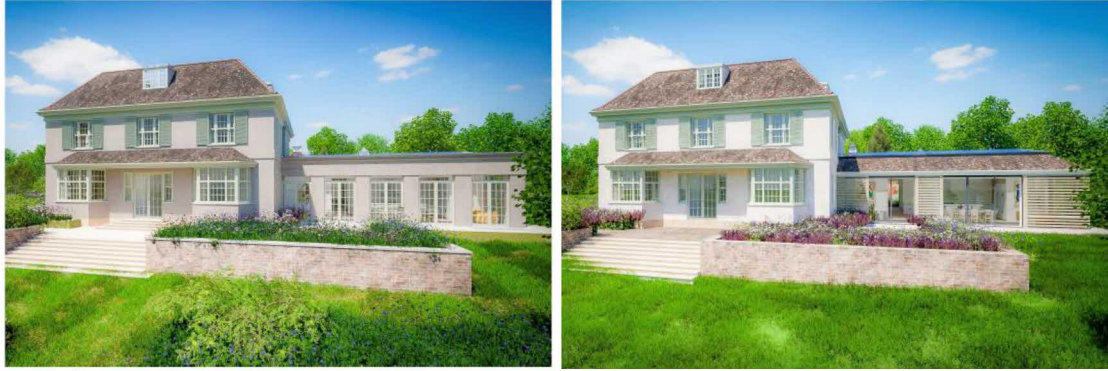
Fig.3 (above left) - Early concept design. A more traditional orangery-style flat roof is concealed behind a parapet. The design creates a greater solid mass and visual draw with contrasting style against the existing, causing more perceived harm to the existing.
