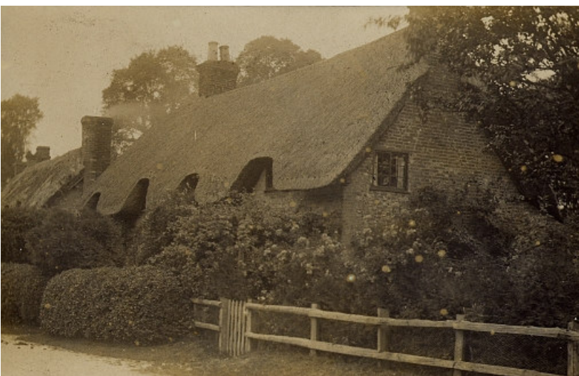
Fig 1949.08A Image dated 1920 showing the gable end of the cottage
