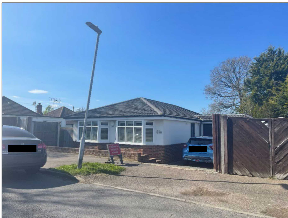
Figure 3: Photograph of 87a Compton Place, following the development of the site.
