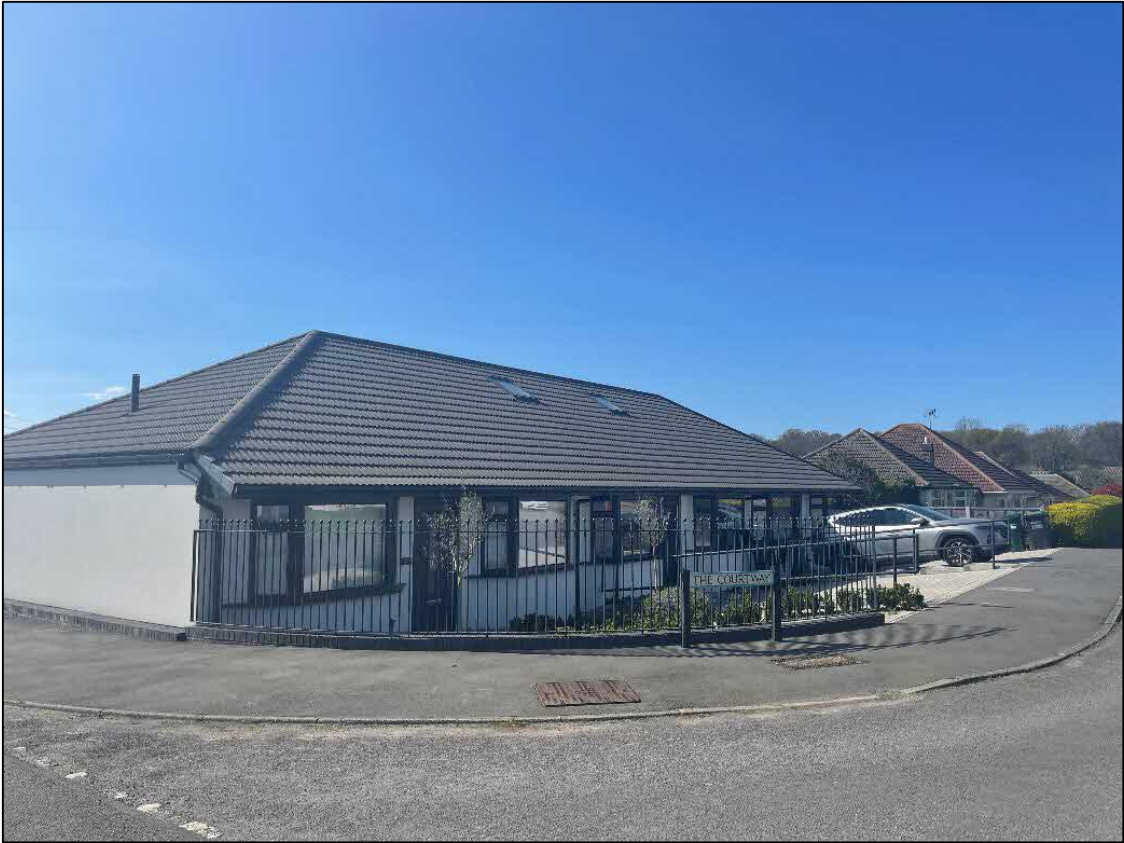
Figure 6: Photograph of 2 The Courtway, following the development of the site.
