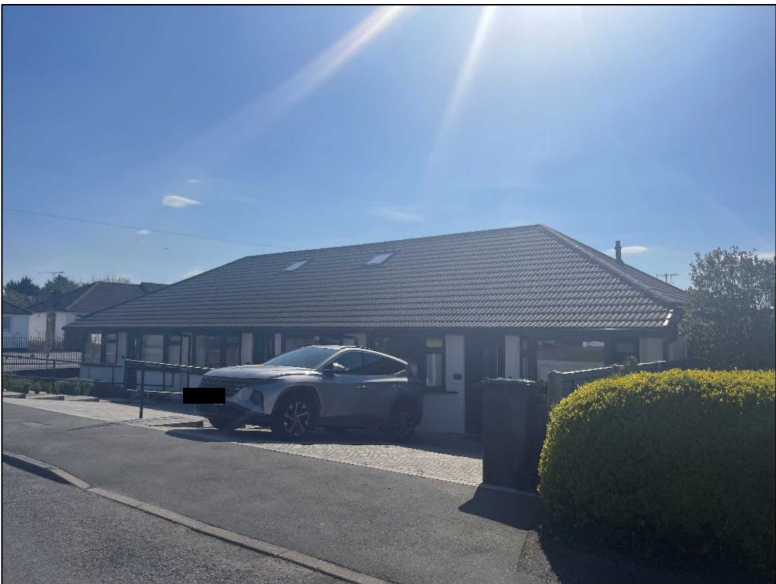
Figure 5: Photograph of 2 The Courtway, following the development of the site.
