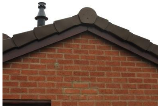
Fig. 13 Sealed gable to the east
