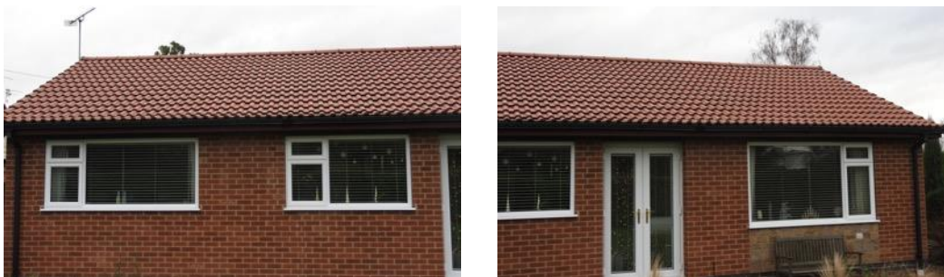
Figs. 6 & 7 Ridge and roof tiles to the southwest
