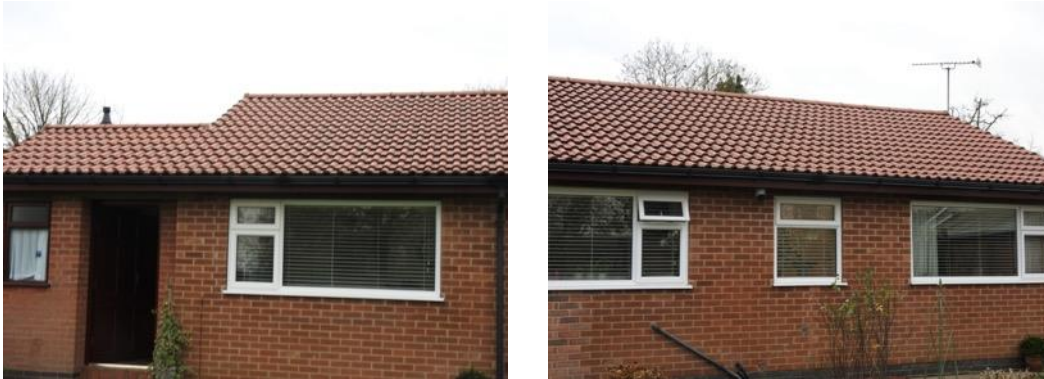
Figs. 9 & 10 Ridges and roof tiles to the northeast
