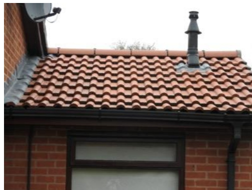
Fig. 8 Ridge and roof tiles to the southwest
