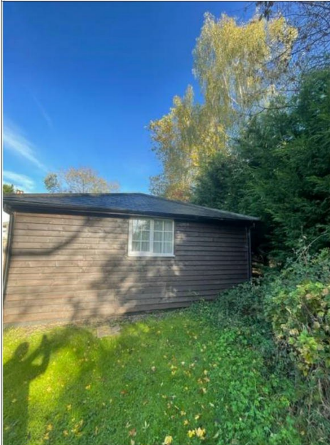
Photograph 11: Side of timber shed.
