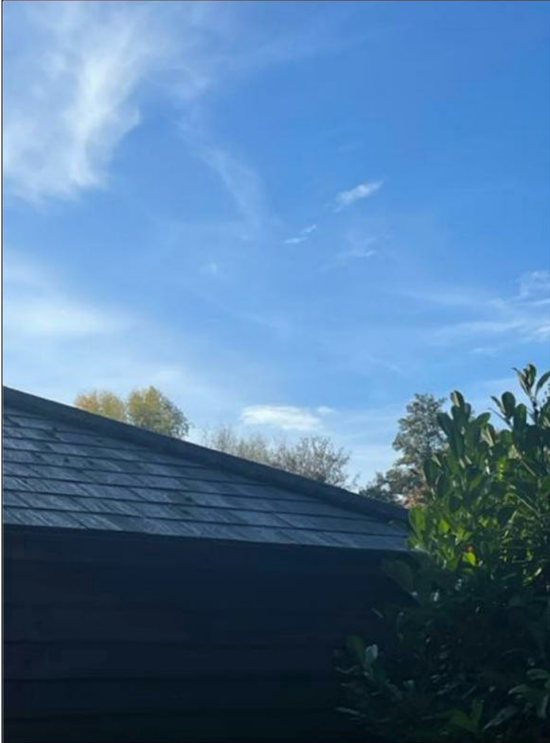
Photograph 21: No gaps under roof tiles.
