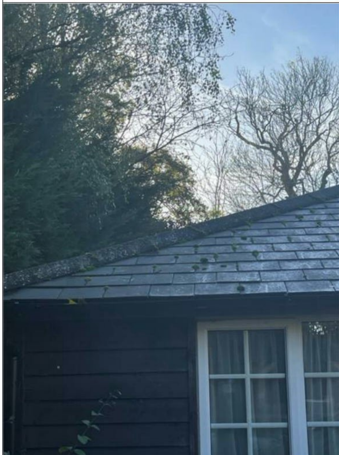
Photograph 19: No gaps under roof tiles.
