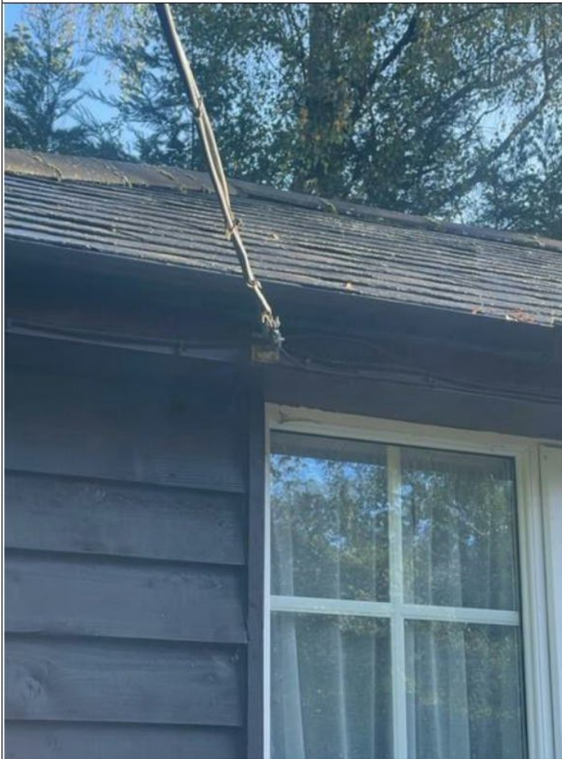
Photograph 3: No gaps around cladding.
