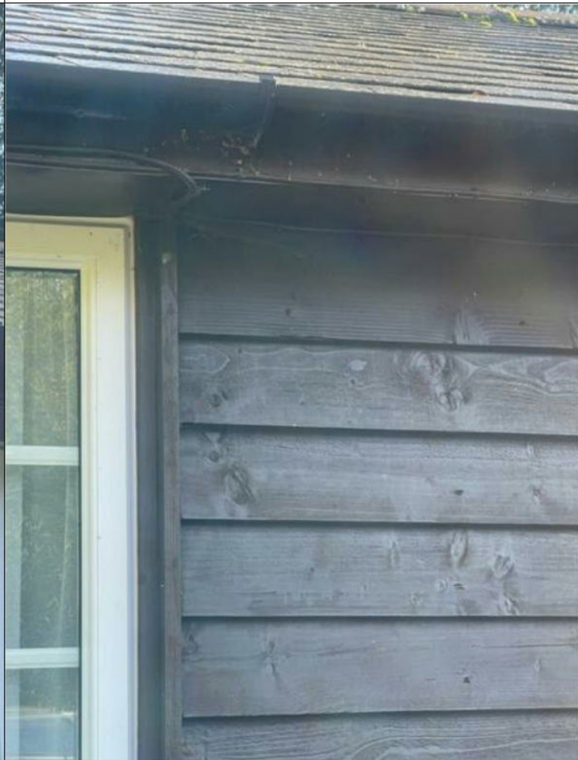
Photograph 4: No visible gaps in cladding.
