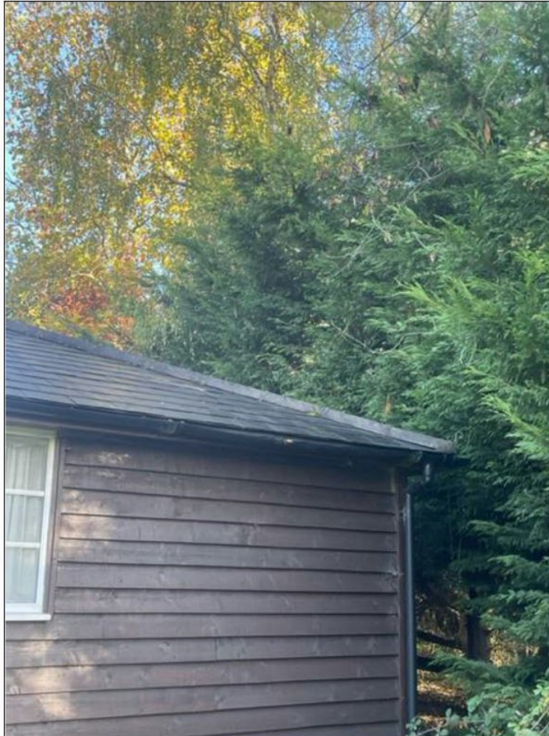
Photograph 13: No gaps in the cladding.
