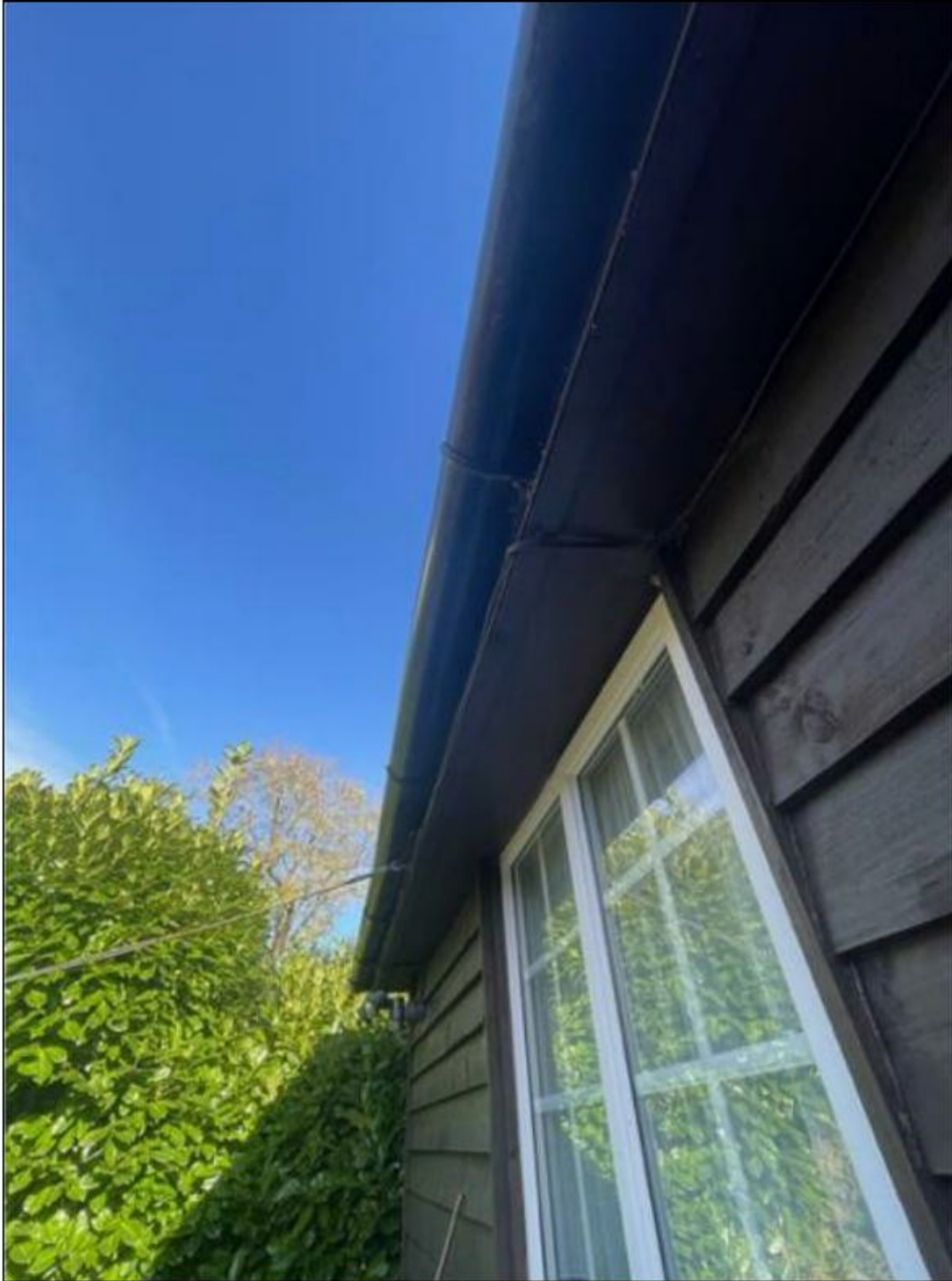
Photograph 5: No gaps in soffits.
