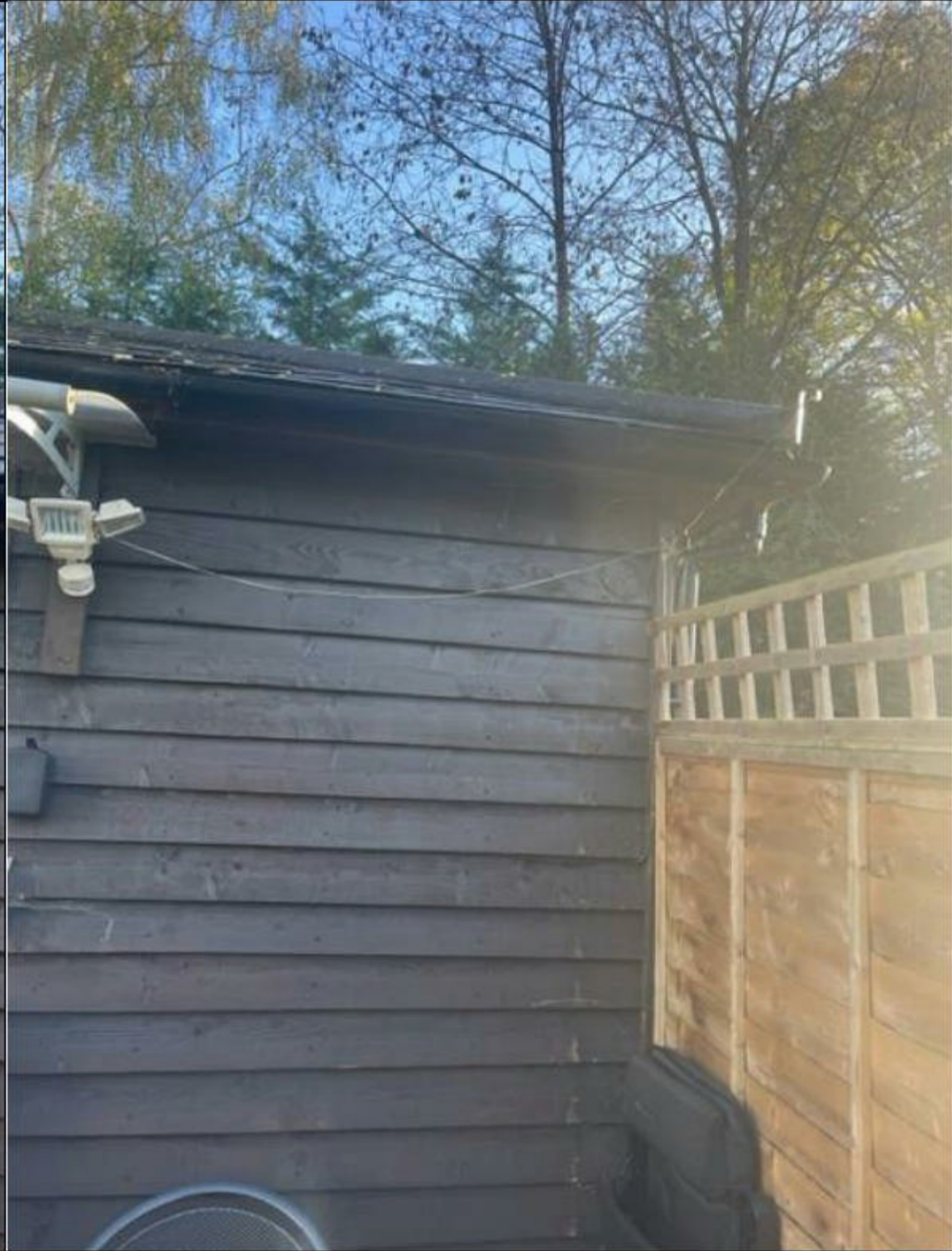
Photograph 10: Tightly constructed cladding.
