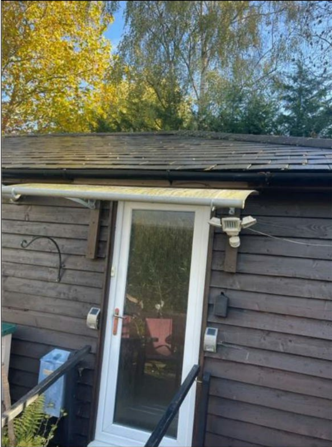
Photograph 9: no gaps in cladding or roof tiles.
