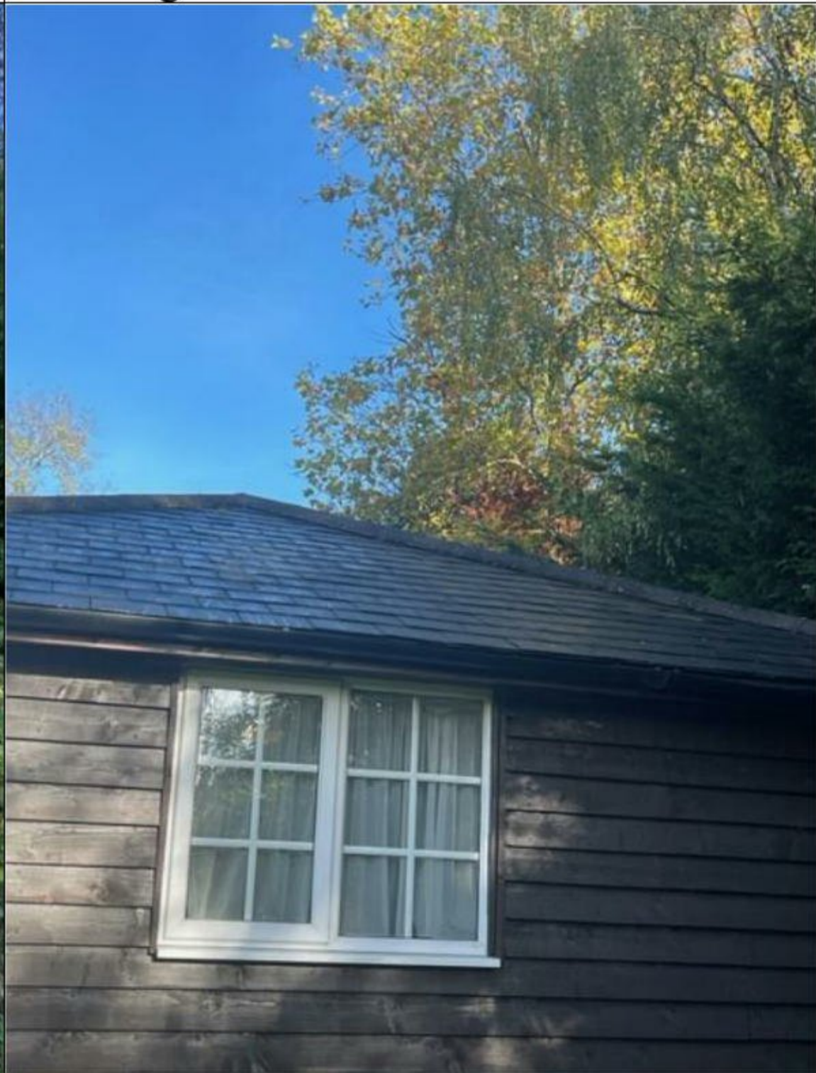
Photograph 12: Side of timber clad shed.
