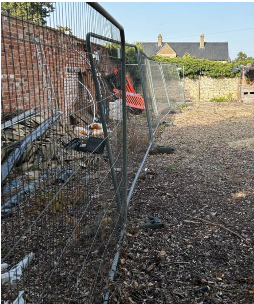
View along west wall
