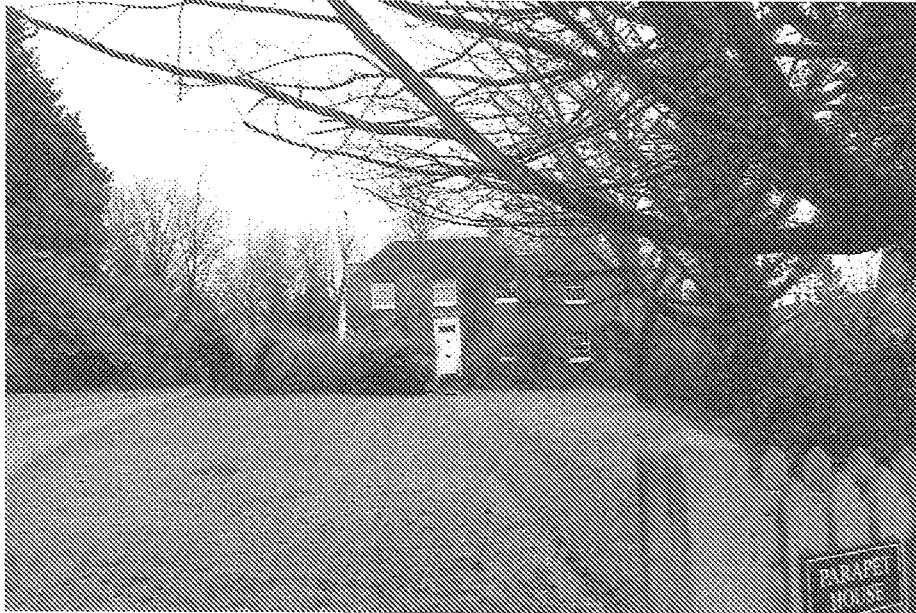
Front View of Parapet House from footpath
