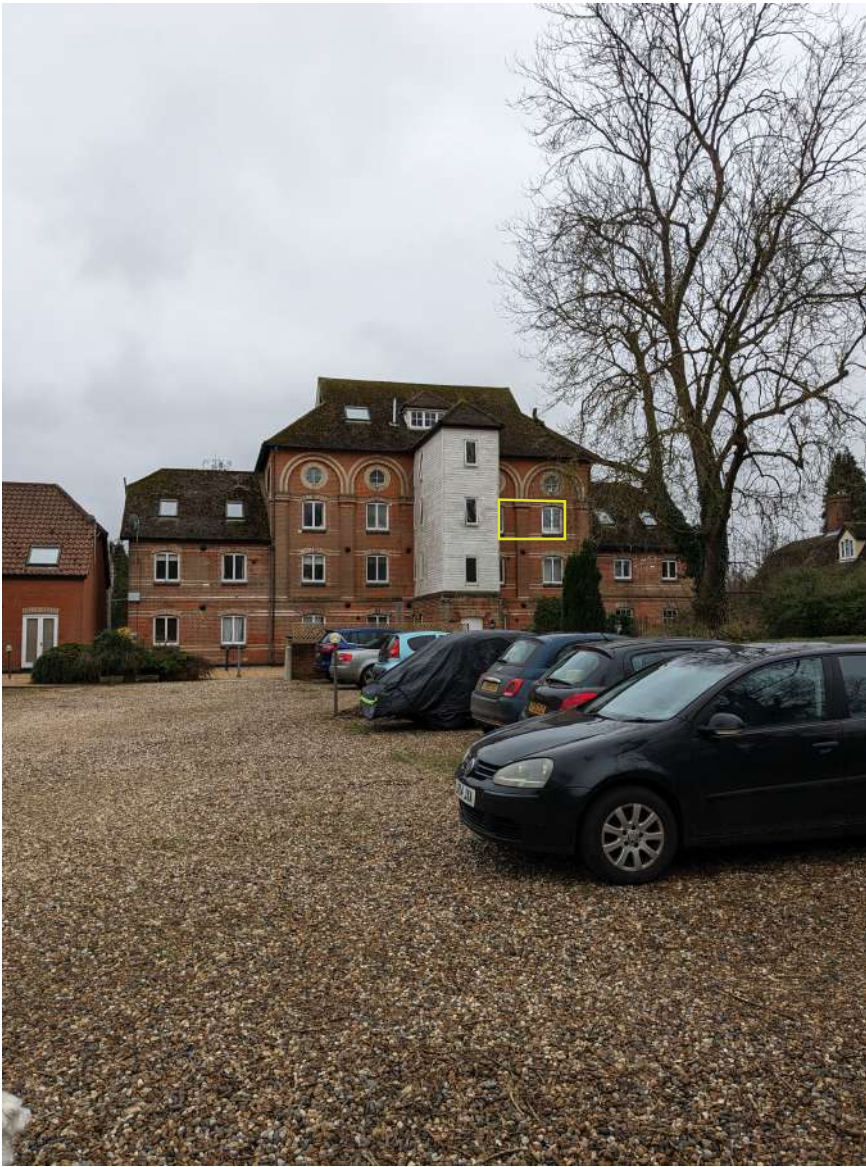
View of the Rear Elevation of Hawks Mill, as seen from Car Park. The two windows serving Flat 6 are highlighted
