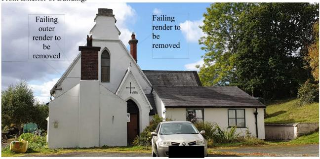
Please note: The render on the labelled part only would be removed, and the original building exposed. The underlying wall appears to be sound and in good condition as far as can be ascertained. This exposed original wall will be painted white to match in with the rest of the building.
