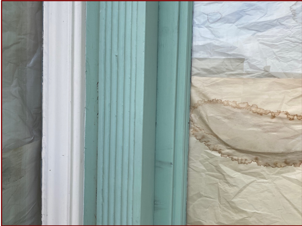
Existing fluted lining to rebated frame.
