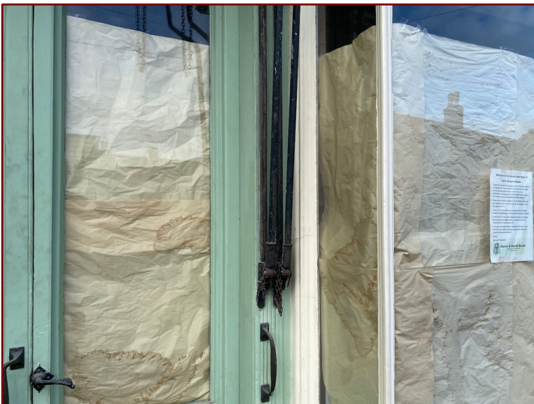
Redundant retractable canopy supports fixed to face of fluted column.
