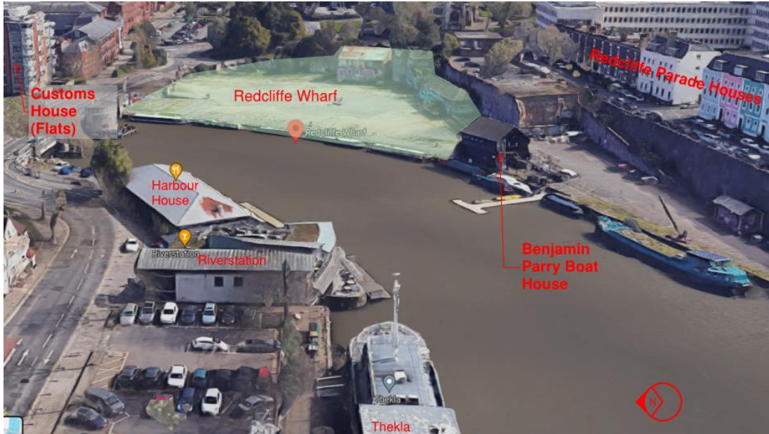
Figure 1 – Existing Site and surroundings. image © Google
